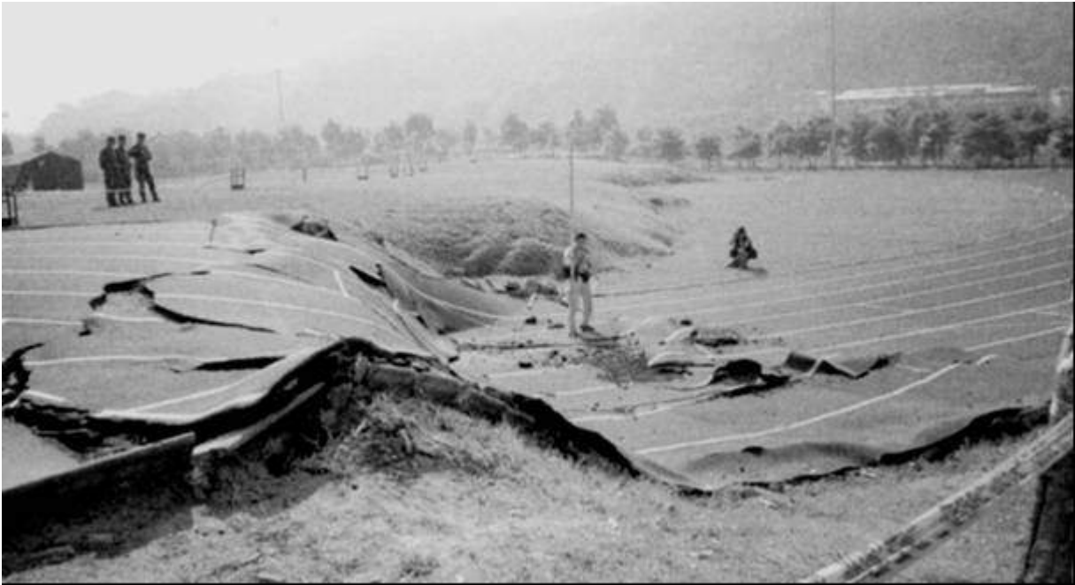
Figure 6.1 Fault scarp formed on the Chelungpu Fault during the magnitude 7.6 Chi-Chi Earthquake, Taiwan, 1999. The disrupted running track shows damage typical of a reverse fault ground-surface rupture, which is well expressed on the brittle surface (note the smoother rupture across grass behind). This location lies on a stream terrace that is younger than the previous rupture event on the fault, so that there was no scarp here before the earthquake. This example illustrates the sorts of effects that can be expected across fault scarps in the Waimate District or Waitaki District the next time any particular fault experiences a surface rupture earthquake. Photo from Kelson et al. (2001).
