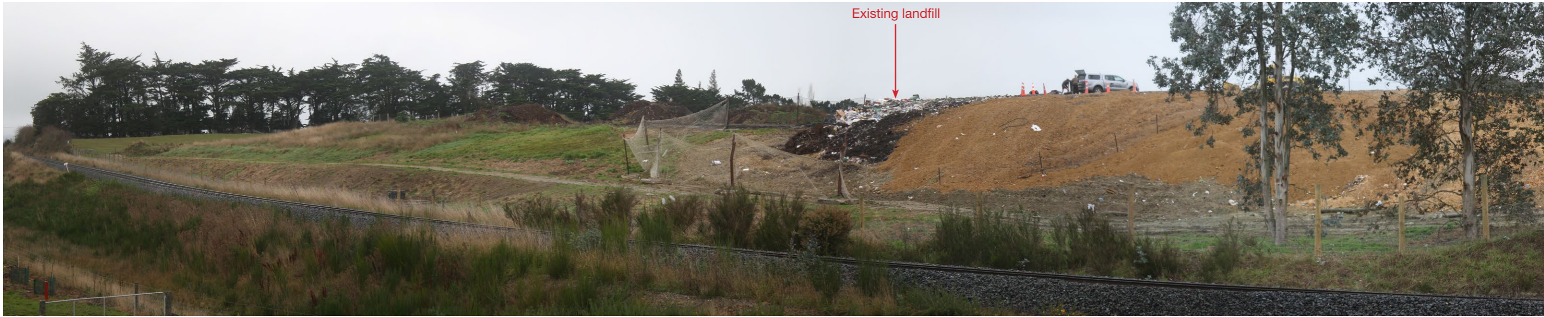
Figure 10: View toward the site from the Balclutha Golf Course, near the railway line
