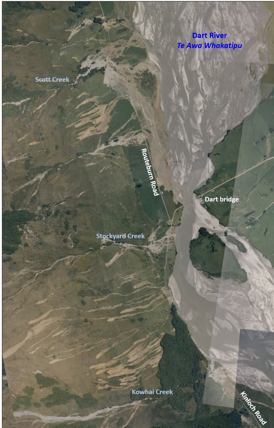
Figure 5.20 January 1994 – disruption to road access and damage to infrastructure and land, caused by flooding of Dart floodplain and alluvial fan and debris flow activity. Includes Scott Creek, Stockyard Creek and Kowhai Creek alluvial fans.
