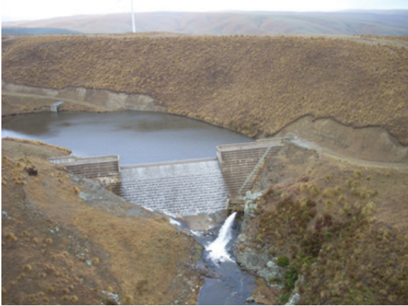
Figure 6.6: RCC Dam – Horseshoe Bend Dam (provided by Pioneer Generation)
