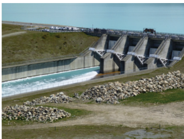
Figure 6.12: Crest Mounted Radial Gates – Pukaki Dam (provided by Meridian Energy)
