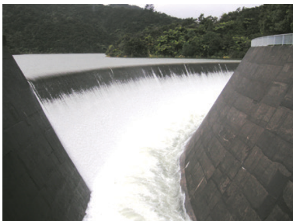
Figure 6.18: Ungated Spillway – Upper Mangatawhiri Dam (provided by Watercare Services)
