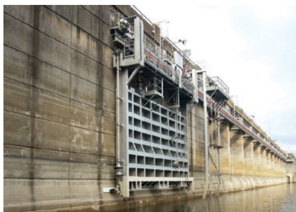
Figure 6.17: Upstream Bulkhead
