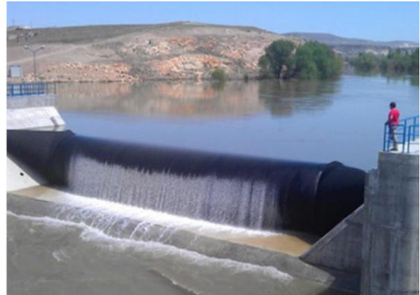
Figure 6.16: Rubber Dam
