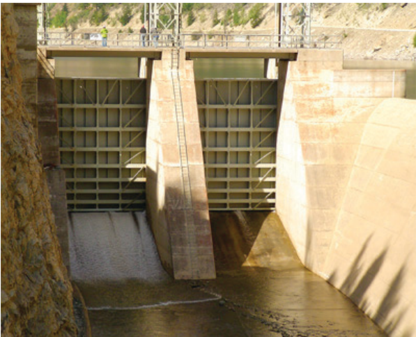
Figure 6.14: Vertical Lift Wheel Gate
