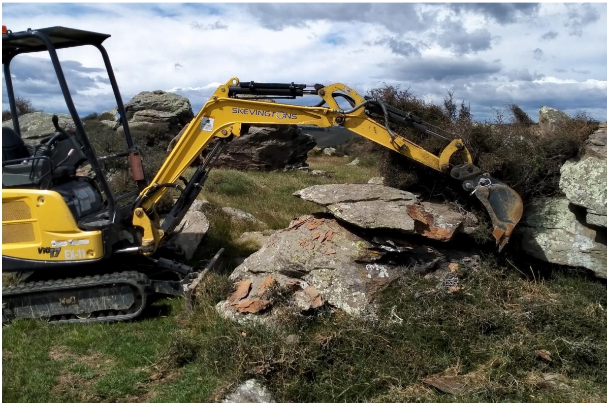
Figure 5.3. Machine-assisted dismantling of a rock tors during the Deepdell North III Project. Image by M. Tocher.
