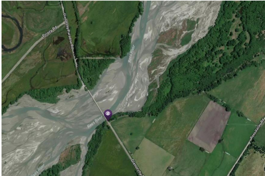
Figure 1. Aerial view of Rees River Bridge
