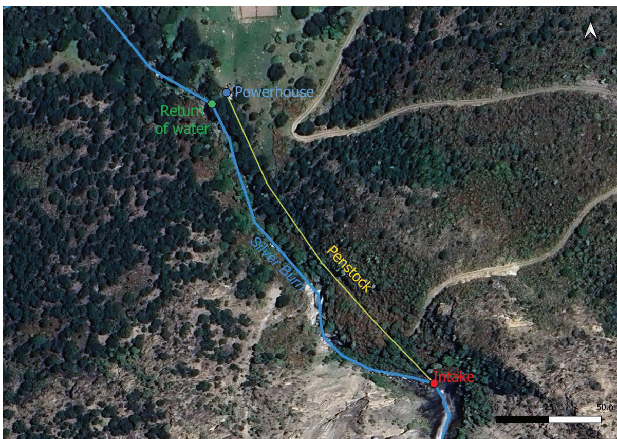
Figure 7 Overview of the Silver Burn Hydroelectricity generation system
