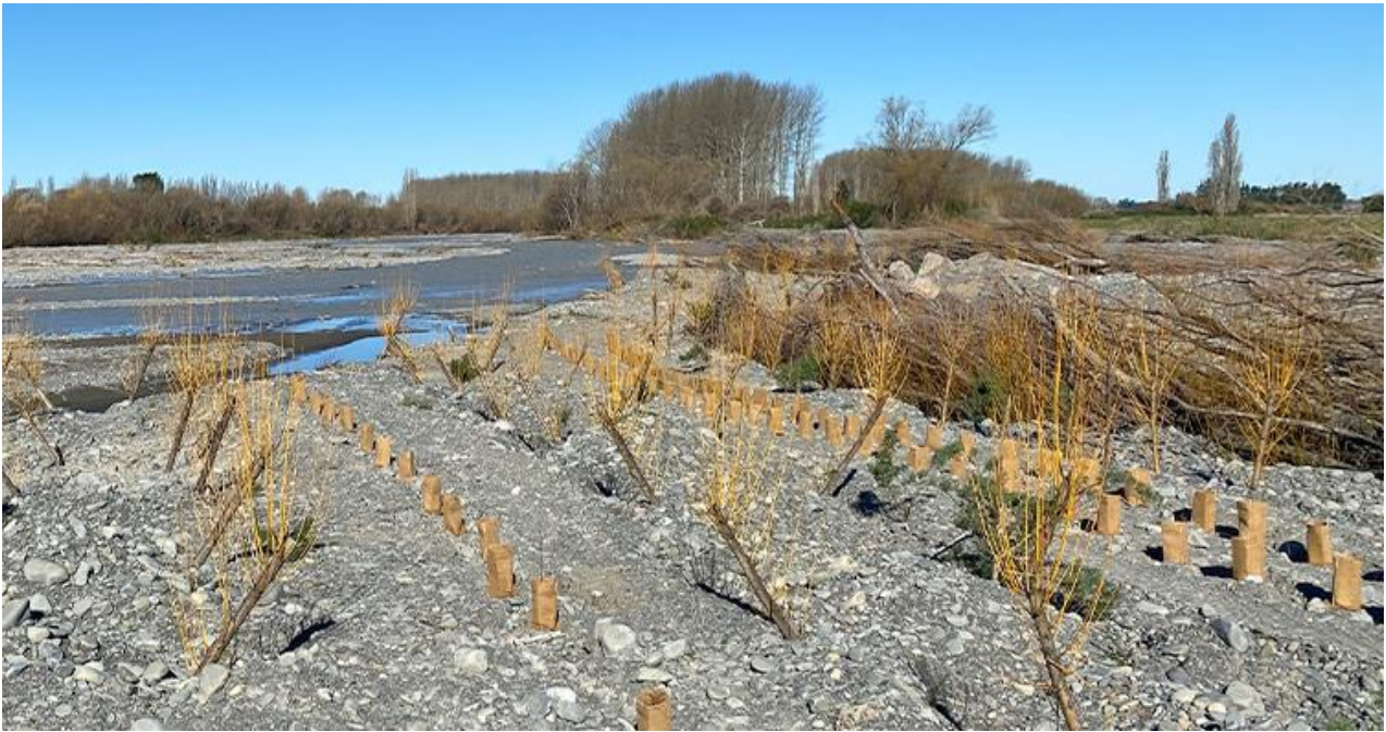
Figure 5.4: Willow pole planting and bioengineered groynes.
