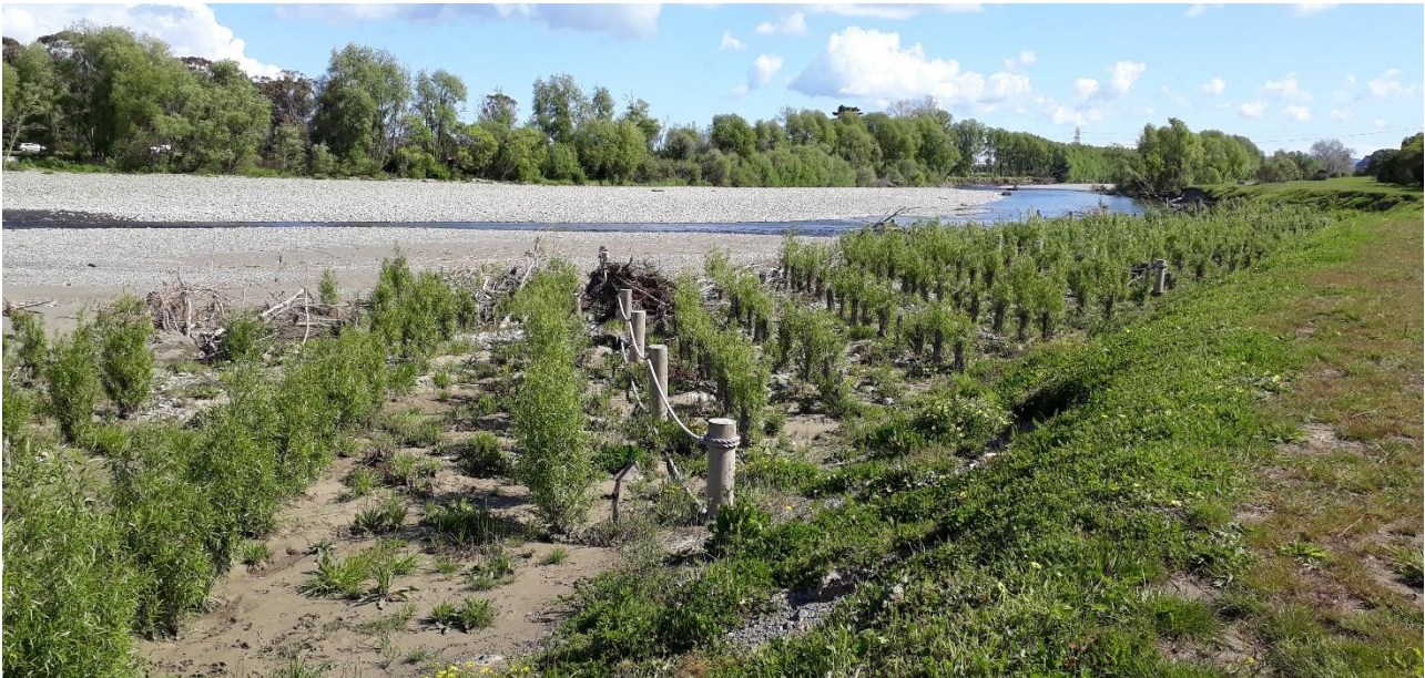
Figure 5.3: Willow pole planting and debris fences made of biodegradable materials.
