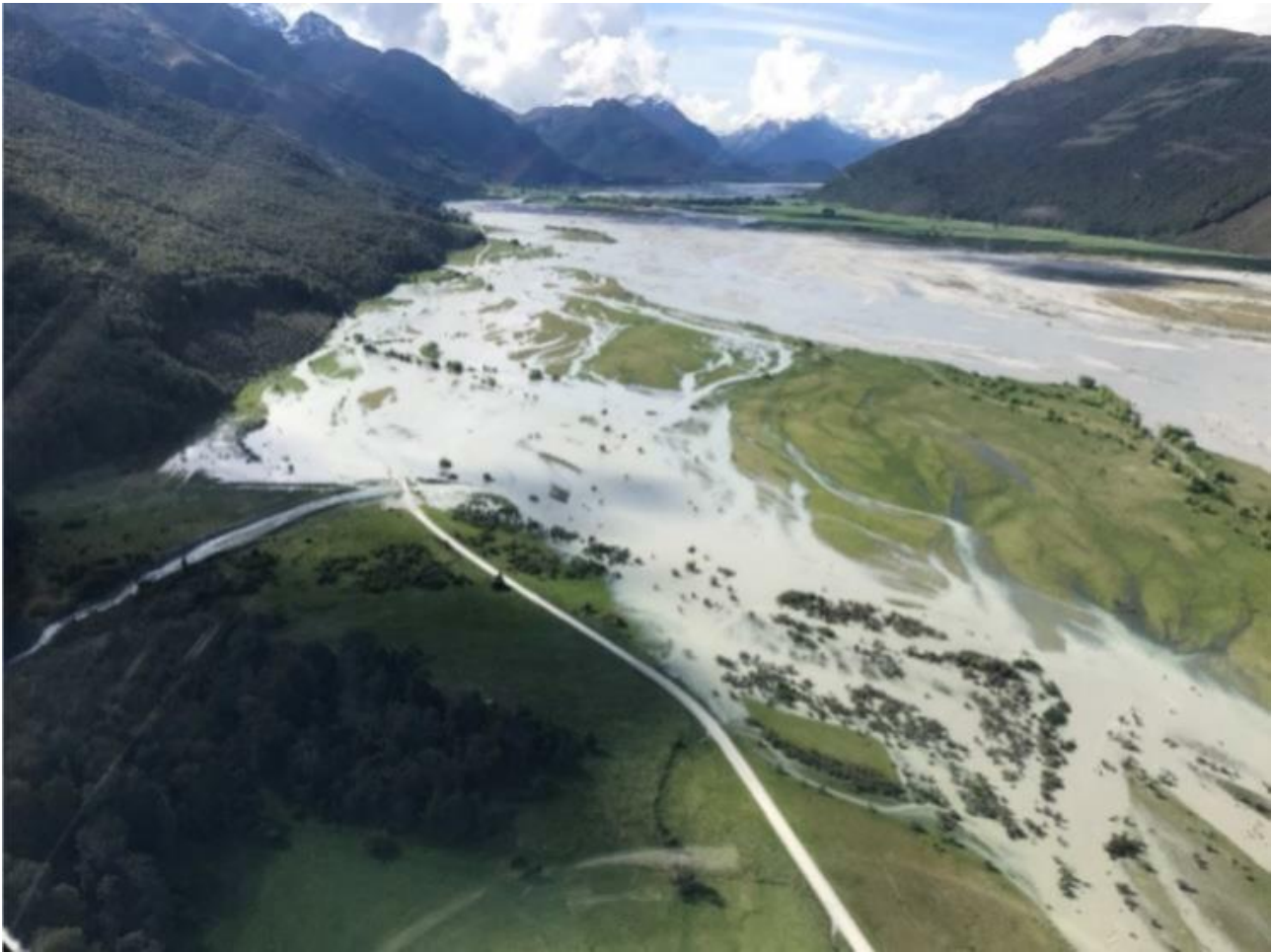
Figure 2.1: Flood inundation of Kinloch Road in a 2019 flood event. Dart River floodplain viewed looking upstream.
