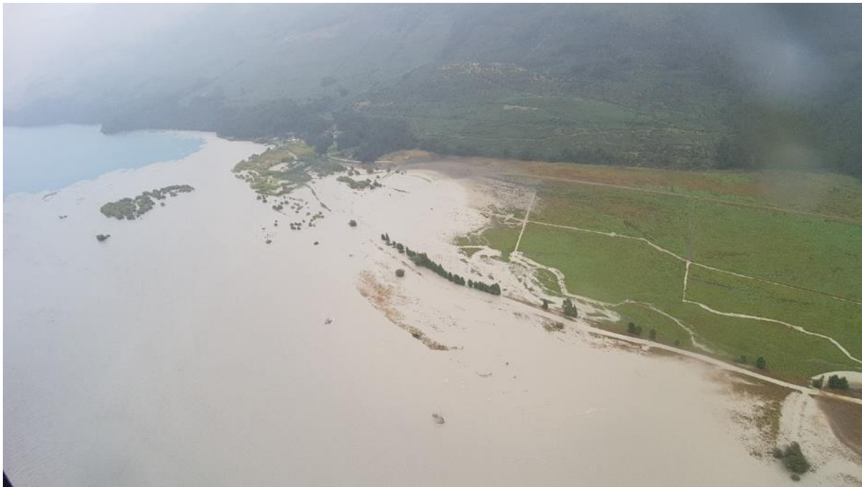
Figure A.5: Aerial view of Kinloch Road flooding during March 2019 flood
