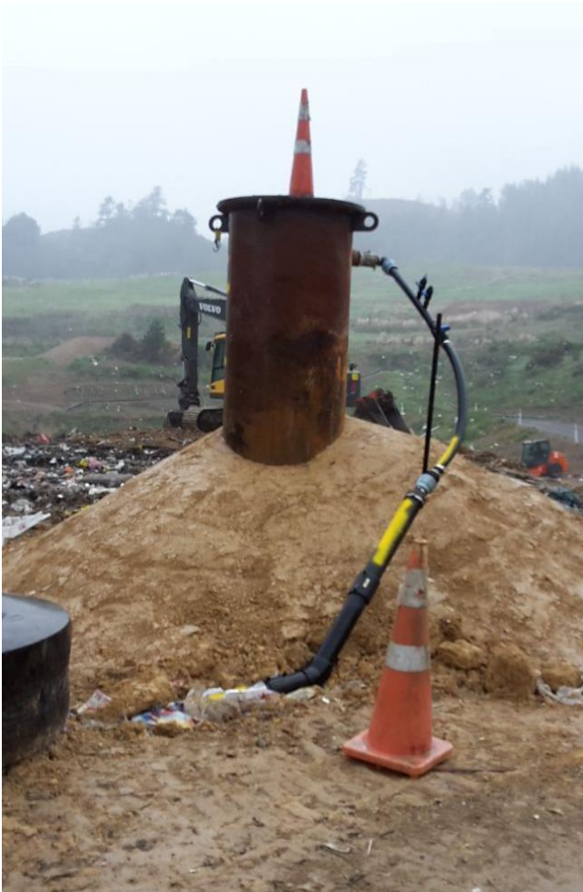
Figure 4.2: Extendable vertical well
