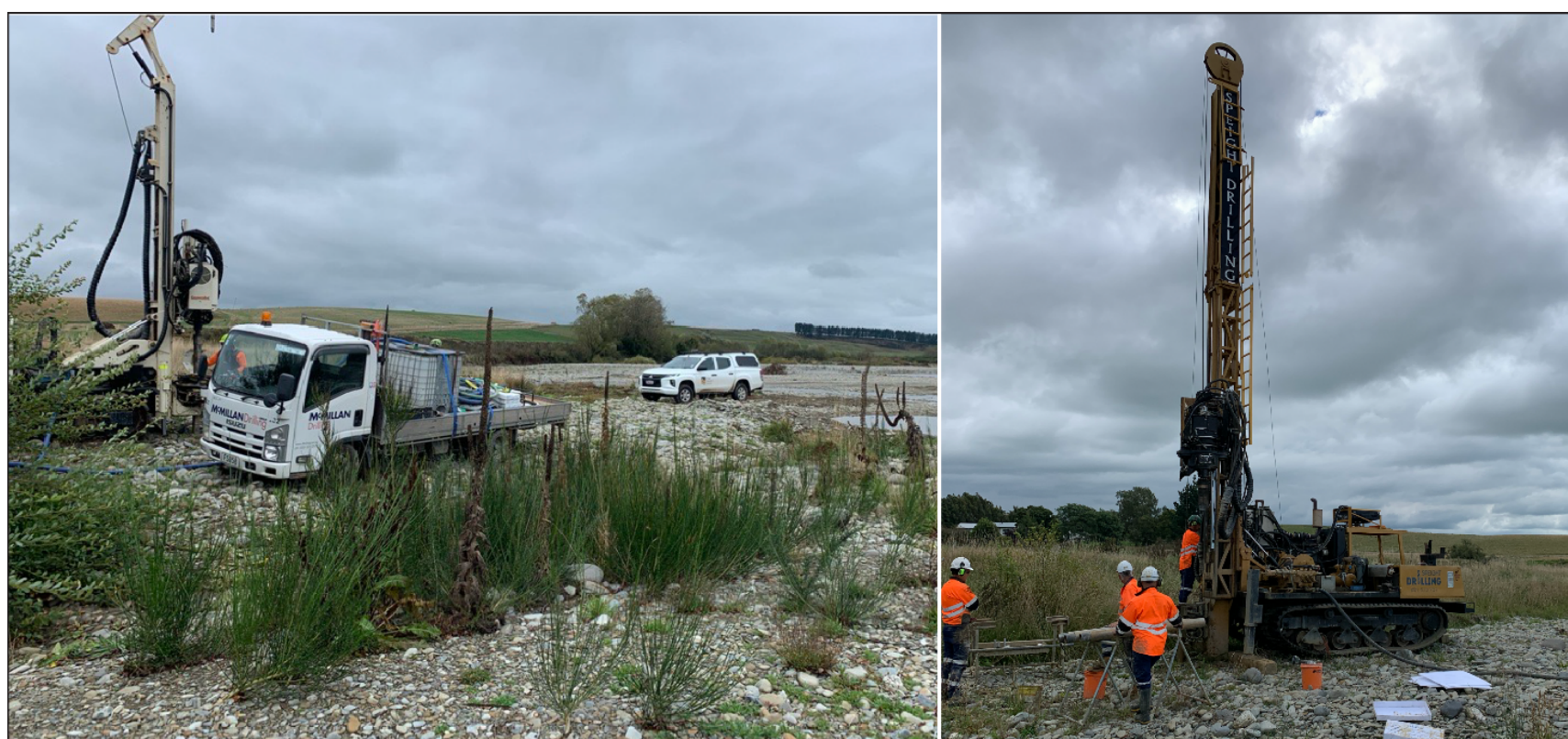
Figure 3. Photos of drilling into the Kauru riverbed at Kininmont Ford.
