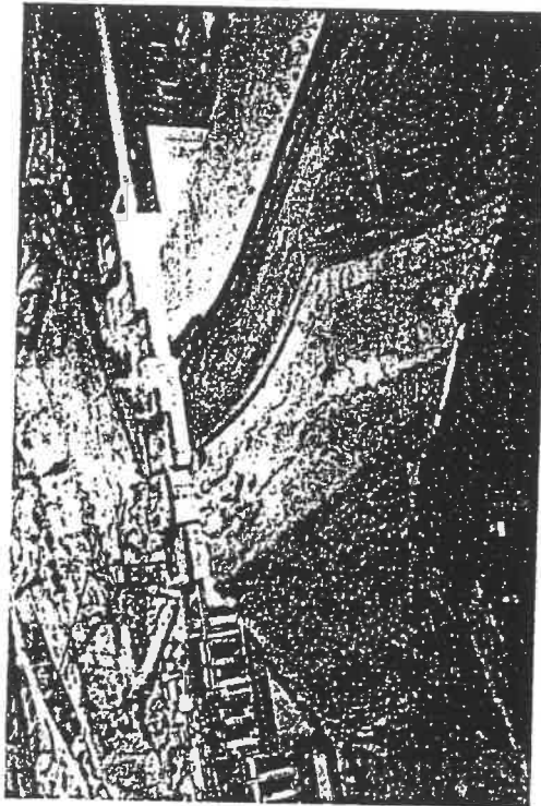
Fig. 4: Compaction of Impervious Clay Core Against Smooth Sloping Concrete Surface with Wheels of Heavy, Rubber-tired Vehicle.
