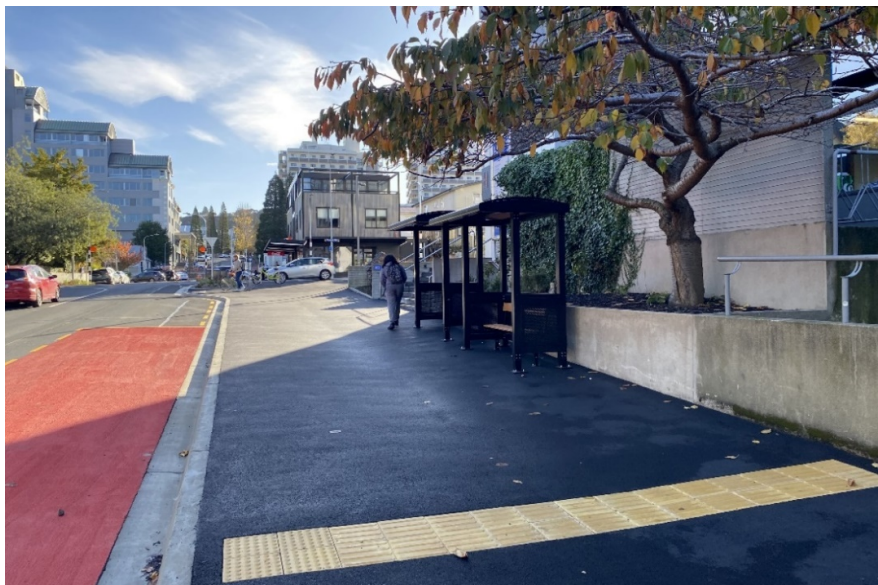
Photo 2: Union Street East Premium bus stop pair (looking west from north side)
