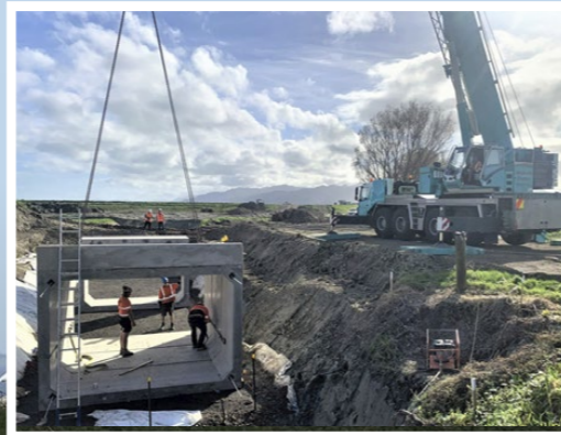
Above: Culvert crossing construction
