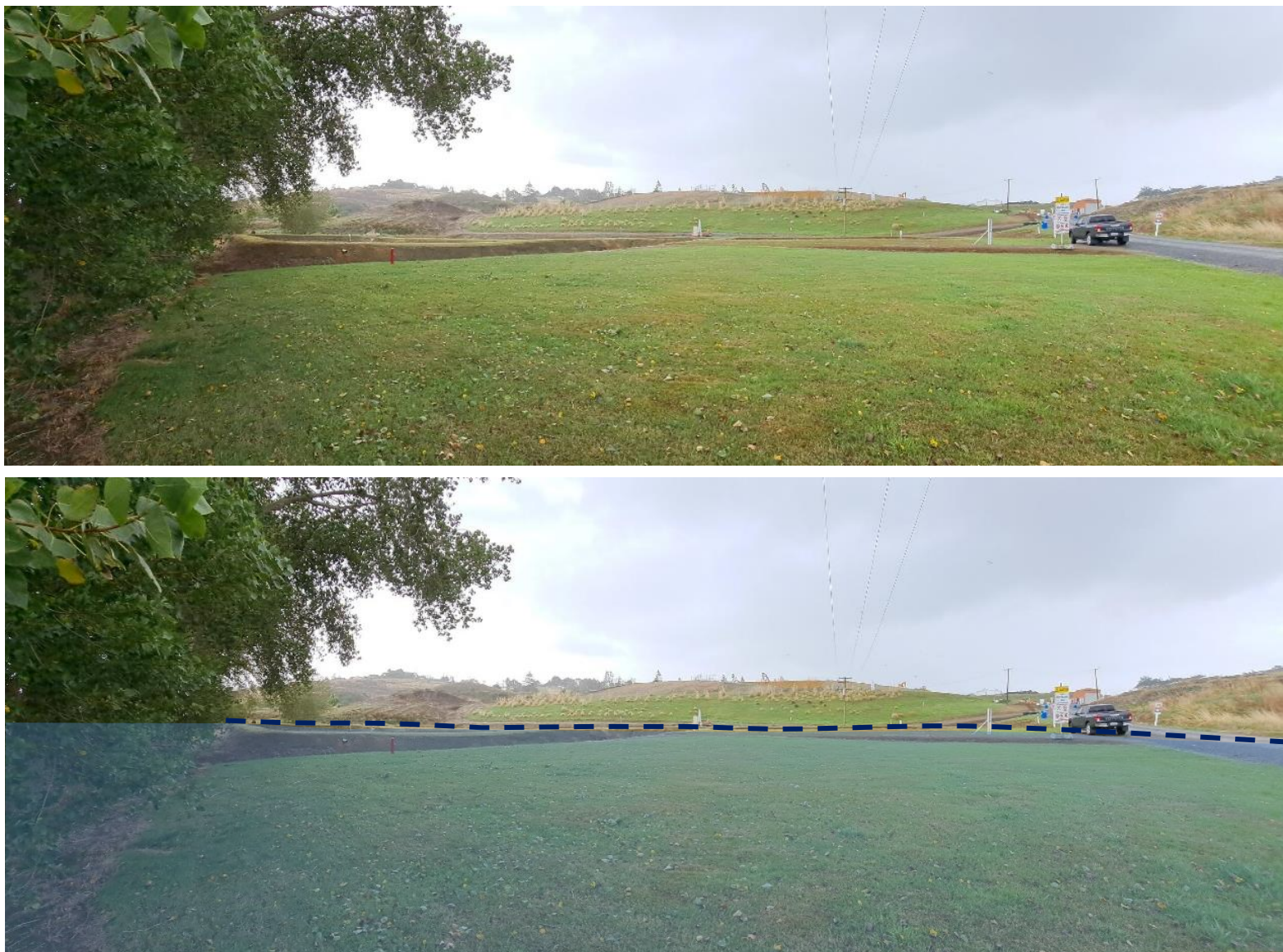
Figure 3-11 Top: view of the berm area and ponds in front of the Mt Cooee landfill. Bottom: showing the boundary of the berm area mapped by GHC.
