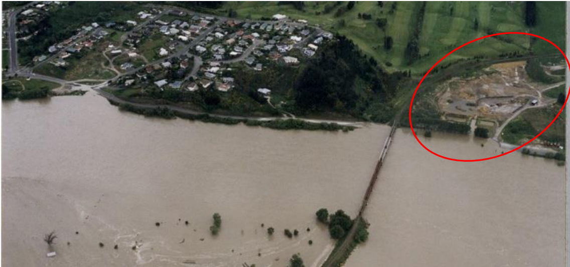
Figure 3-4 View of the Mt Cooee landfill looking north during the November 1999 flood. Source: ORC.
