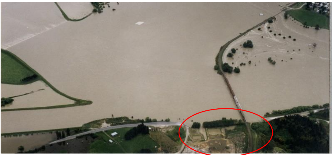
Figure 3-5 View of the Mt Cooee landfill looking south during the November 1999 flood. Source: ORC.
