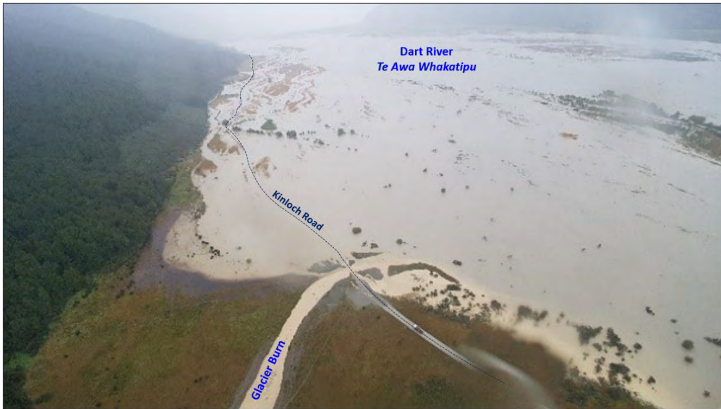
Figure 5.18 March 2019 – flooding of Dart floodplain, showing inundation of Kinloch Road.
