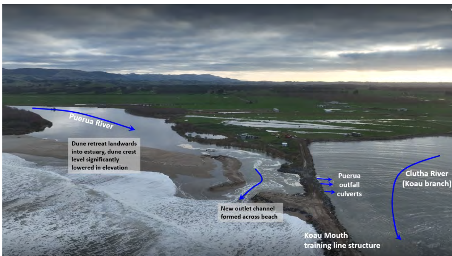
Figure 7: The function of the Puerua Estuary and Lower Clutha Flood Protection and Drainage Scheme following the 2023 event.
