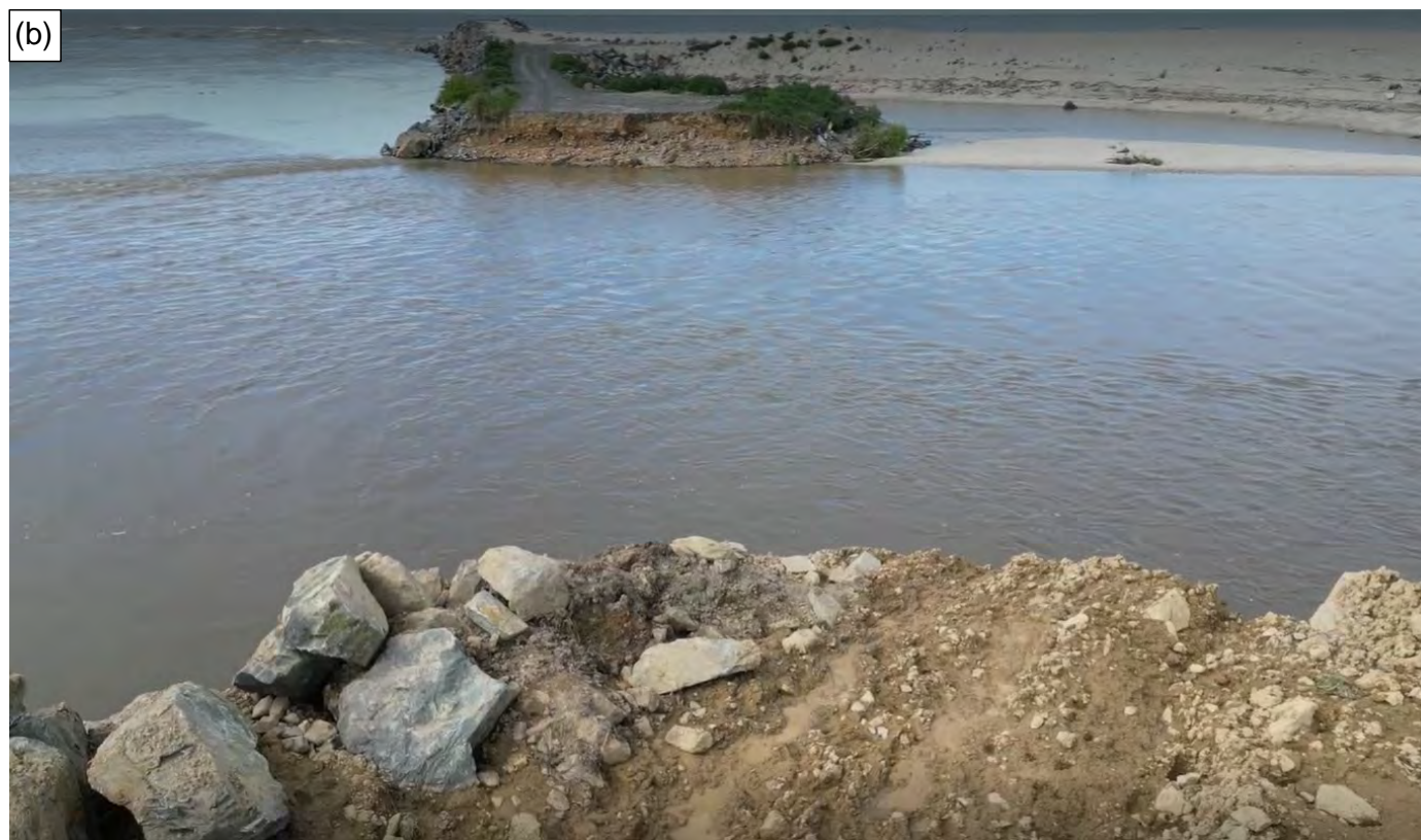
Figure A-1: (a) Flow across access track to Puerua Training Line, and (b) washed out training line following cut and development of wider breach.
