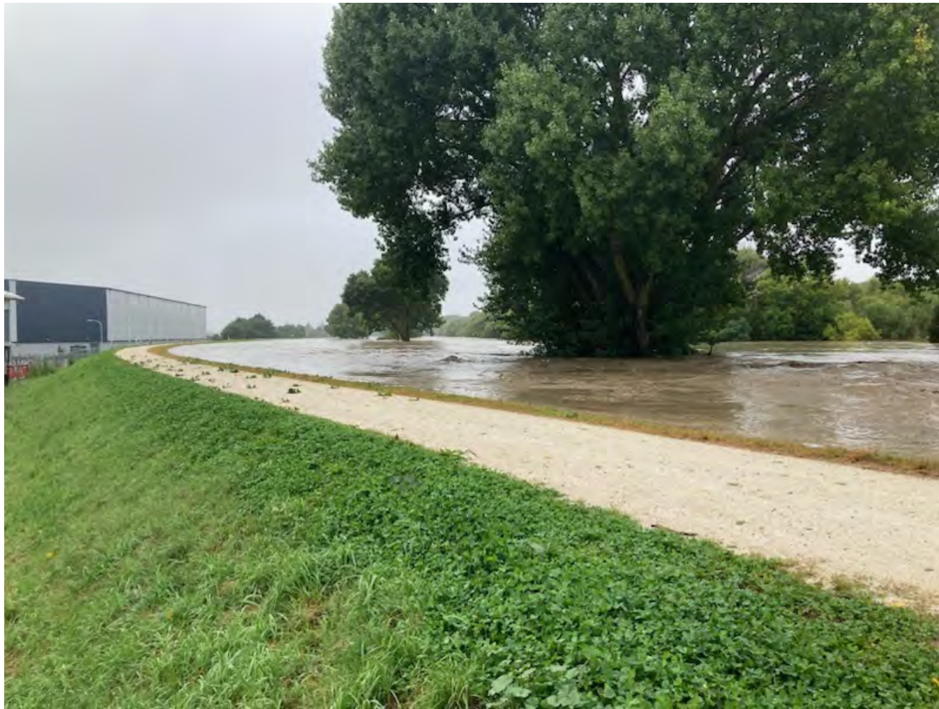
Figure 1: Taradale Stop Bank, Hawkes Bay showing SUP and floodwaters during the 2023 Cyclone Gabrielle event
