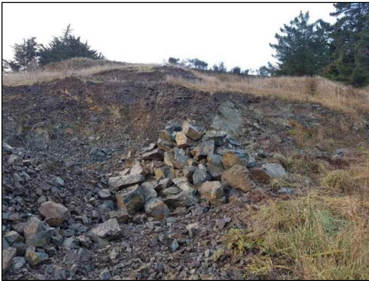
Figure 8: View of cut slope at Site 2
