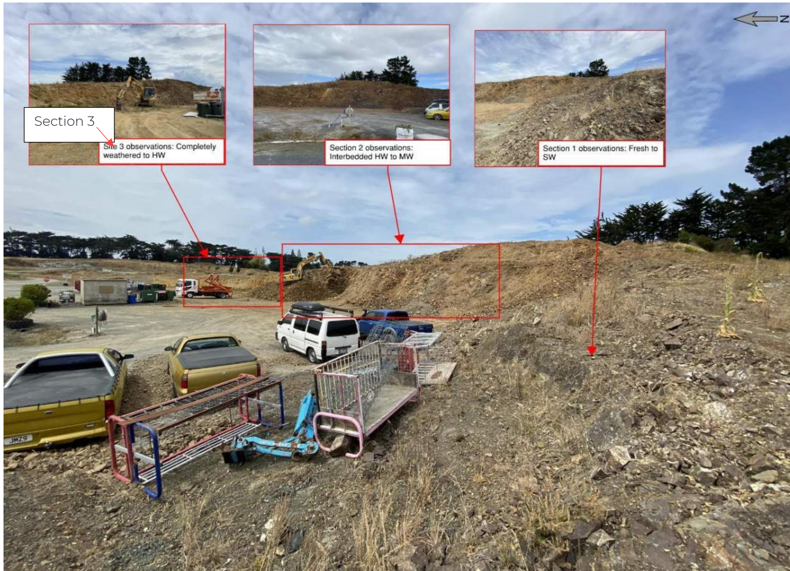
Figure 9: Photograph showing various sections of the cut slope
