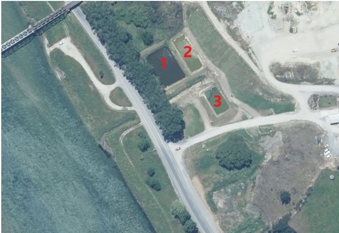
Figure 12 Stormwater retention ponds (1, 3) and leachate emergency overflow pond (2). Source: Otago Maps.
