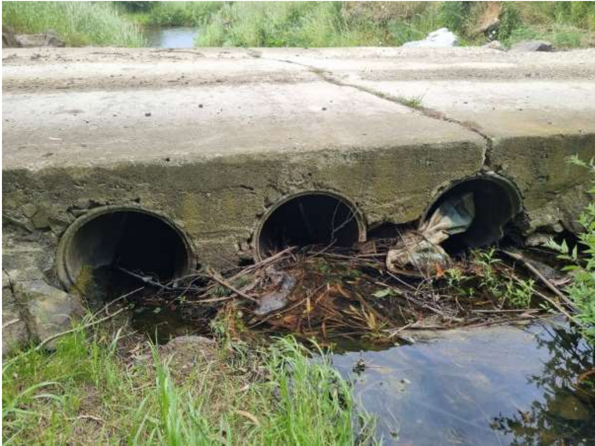
Figure 42 Upstream view of the H1 culverted ford
