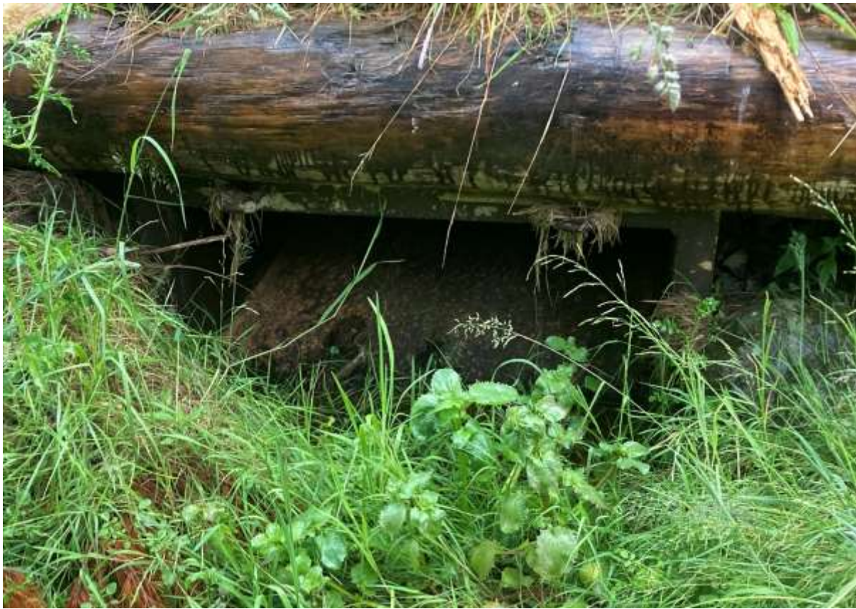
Figure 72 Downstream view of the H11 culvert.
