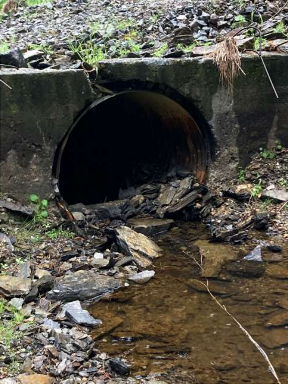
Figure 66 Downstream view of the H9 culvert
