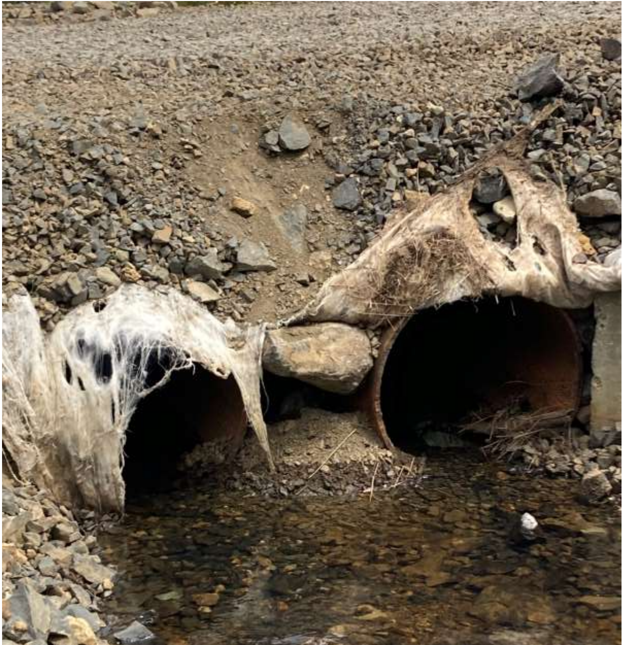
Figure 45 Downstream view of H2 culverts on December 13 th 2023
