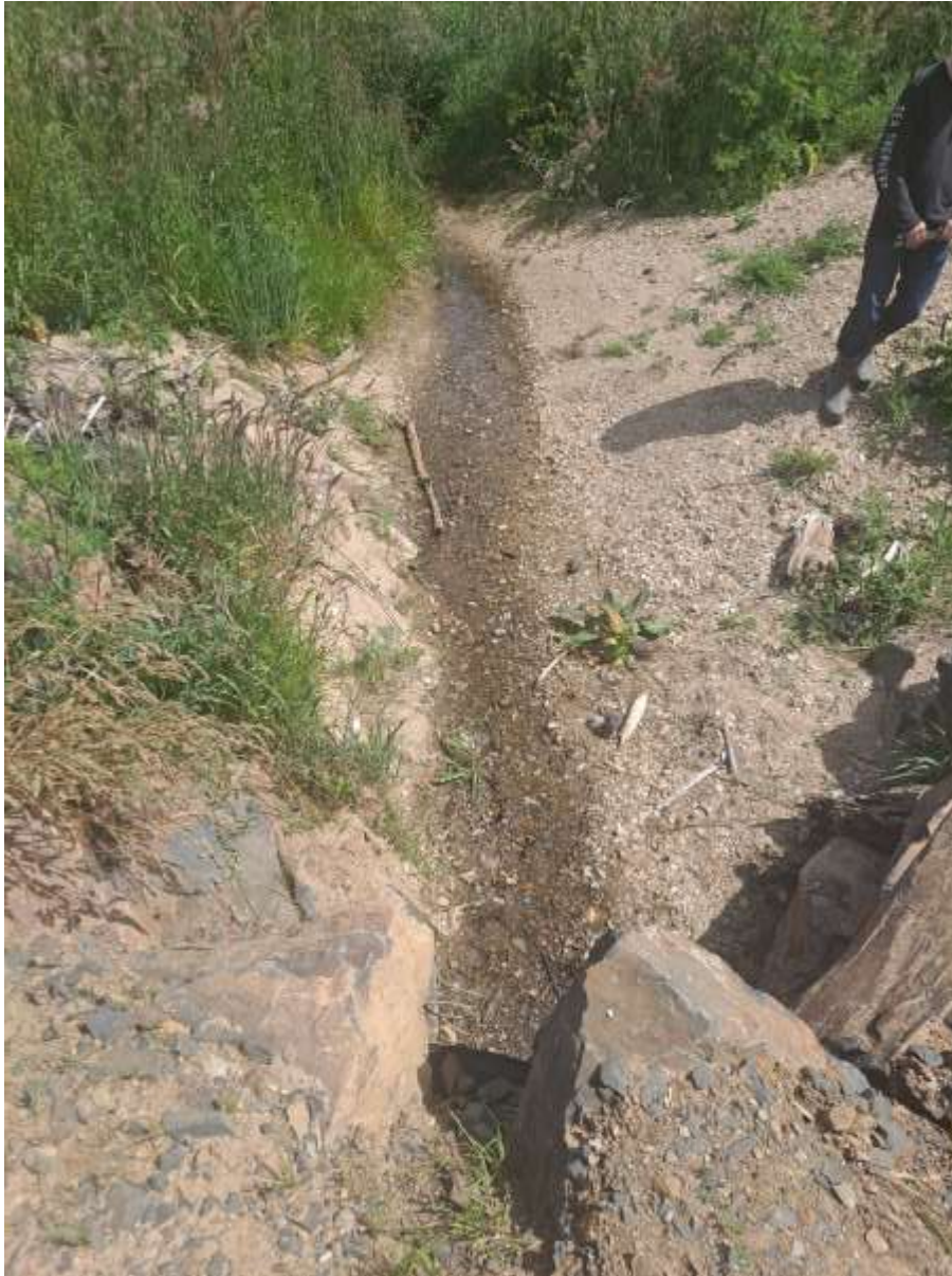
Figure 64 Upstream view from the H8 Culvert
