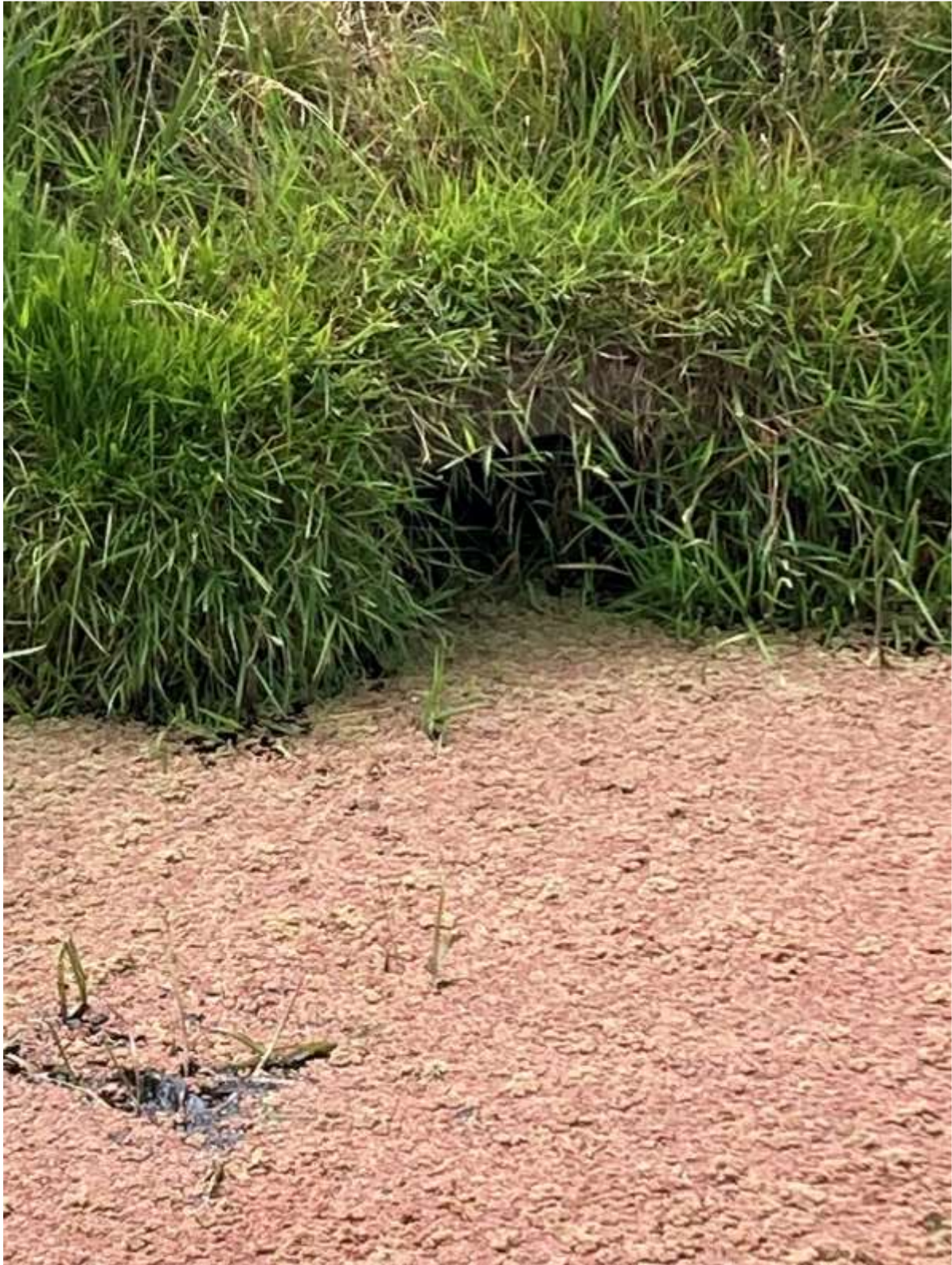
Figure 26 Upstream view of E5 culvert
