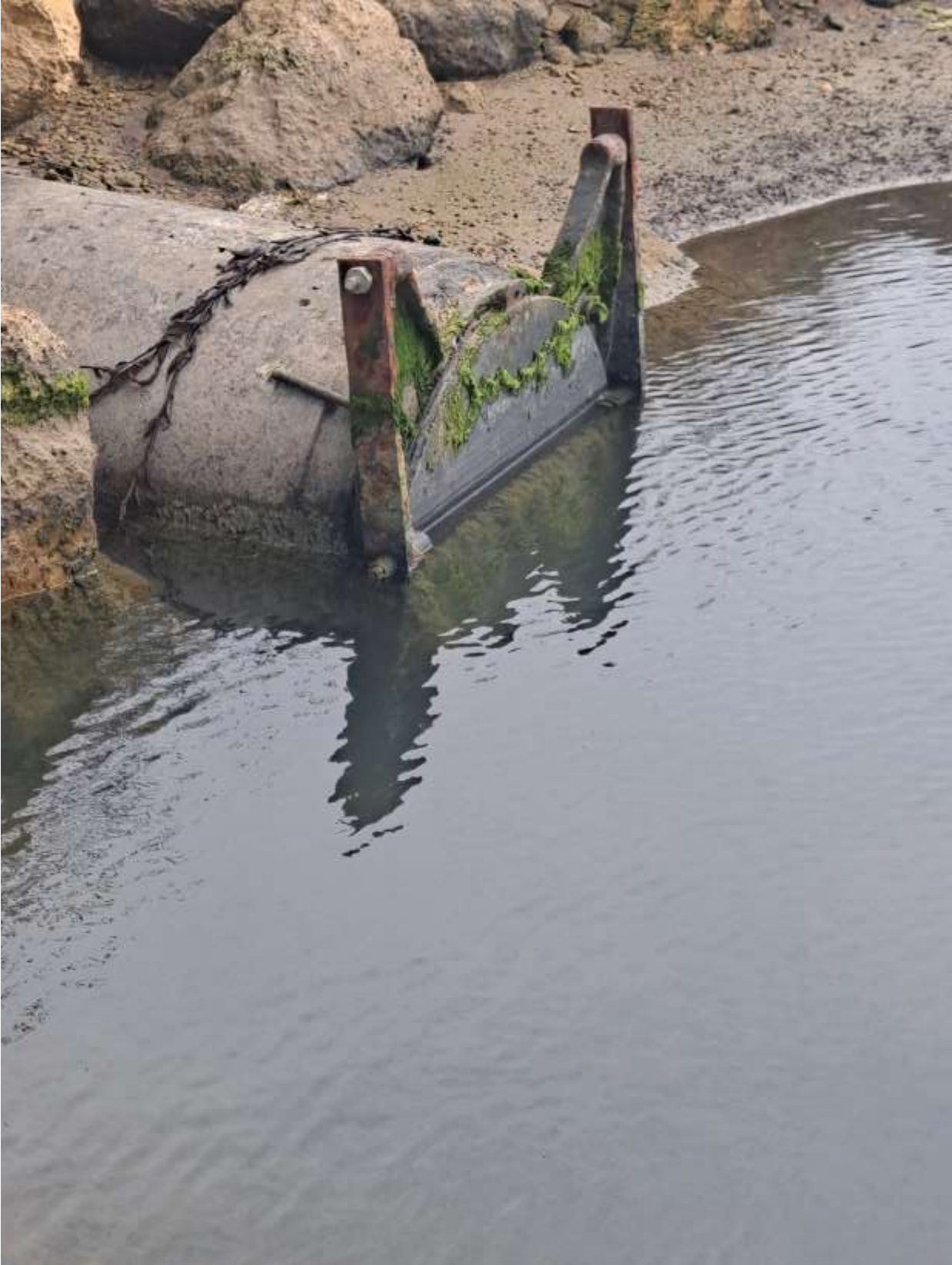
Figure 21 Downstream view of the E3 flap gate
