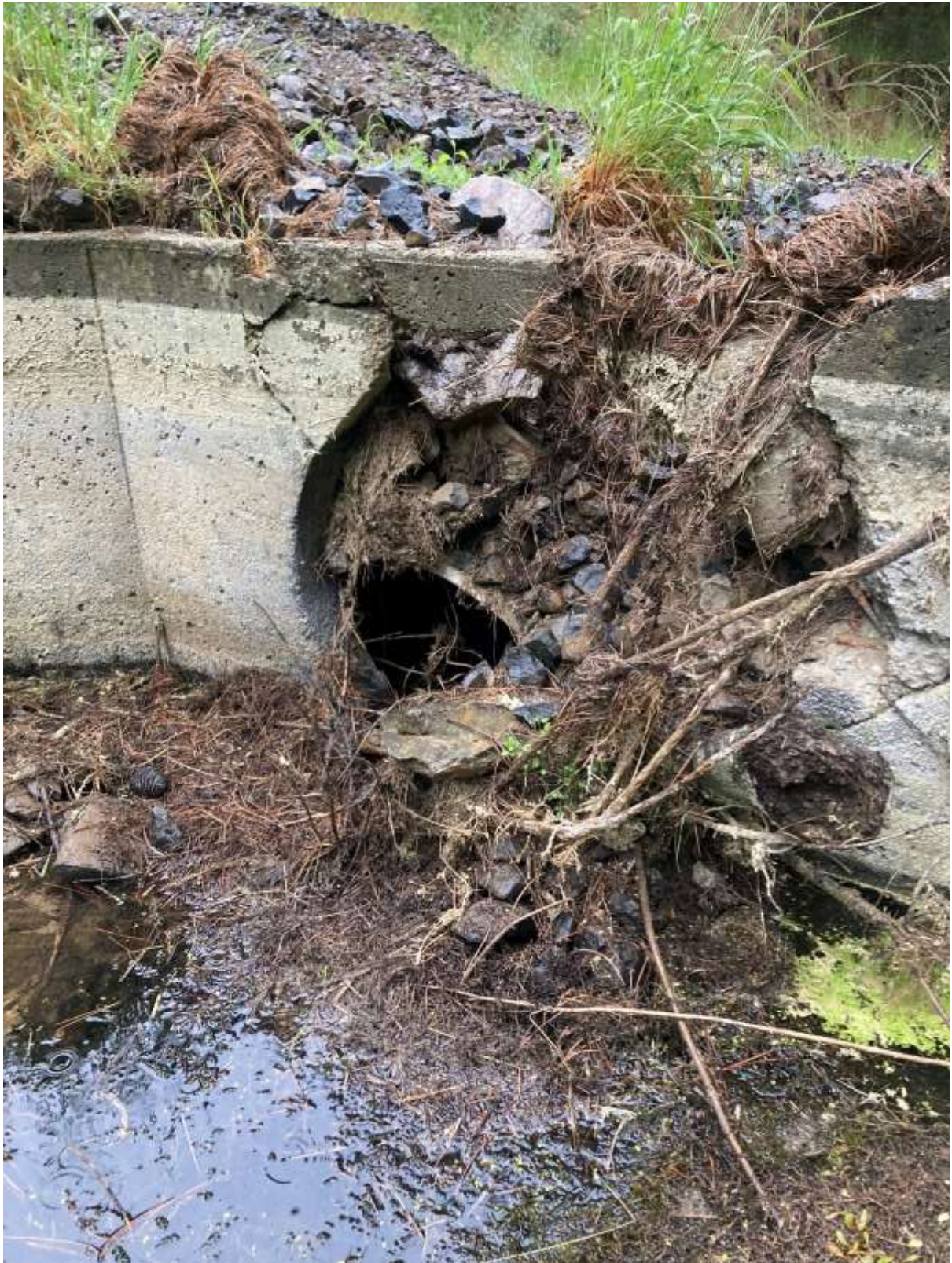
Figure 67 Upstream view of the H9 culvert
