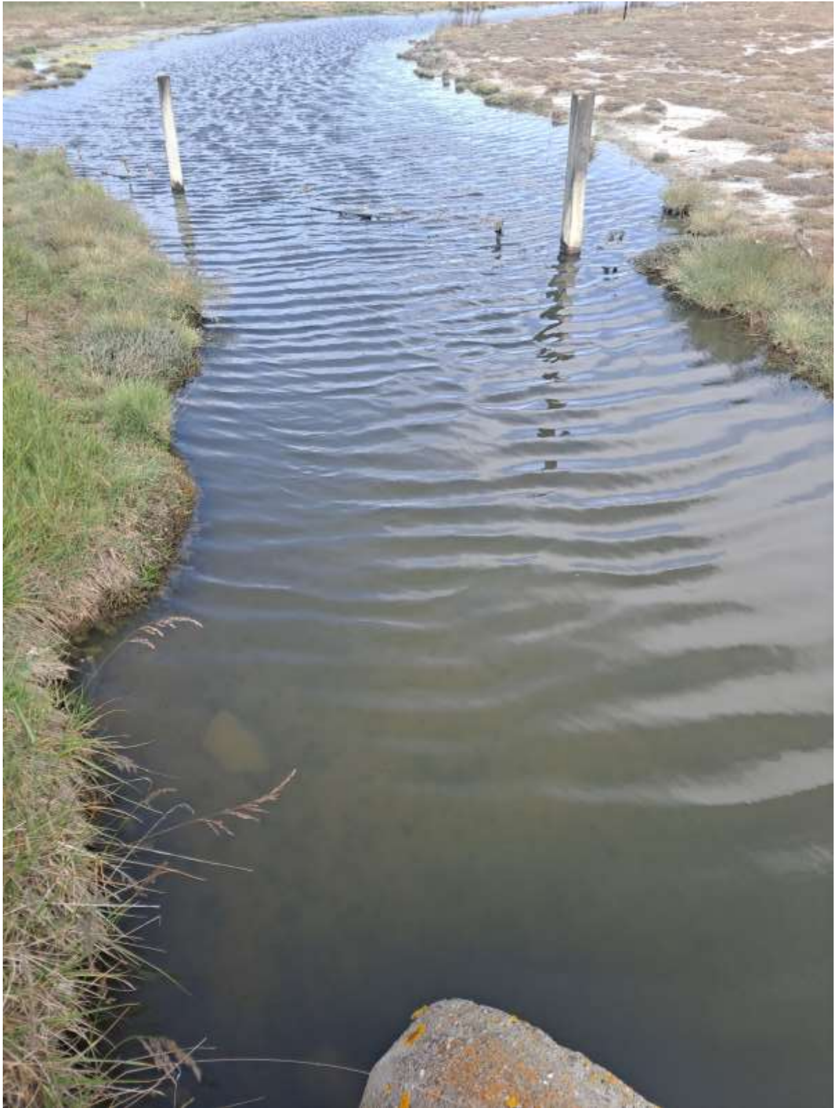
Figure 22 Upstream view of the E3 culvert
