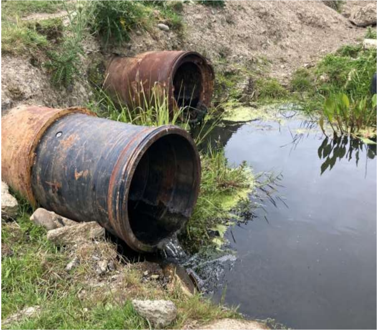
Figure 57 Downstream view of the H6 culverts.
