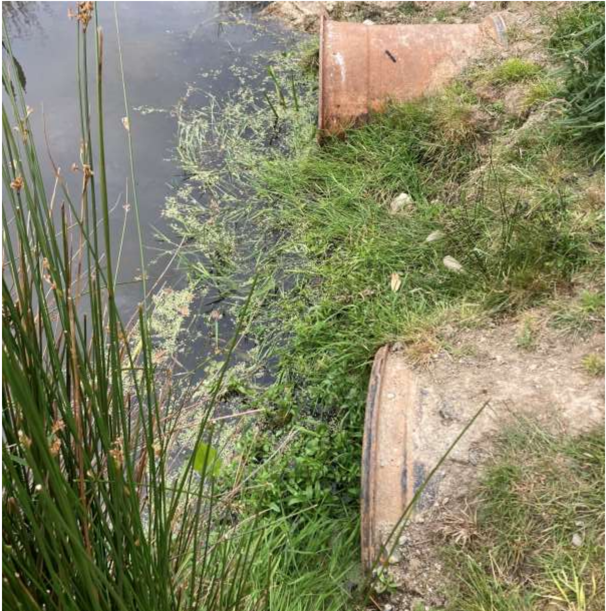
Figure 58 Upstream view of the H6 culverts.
