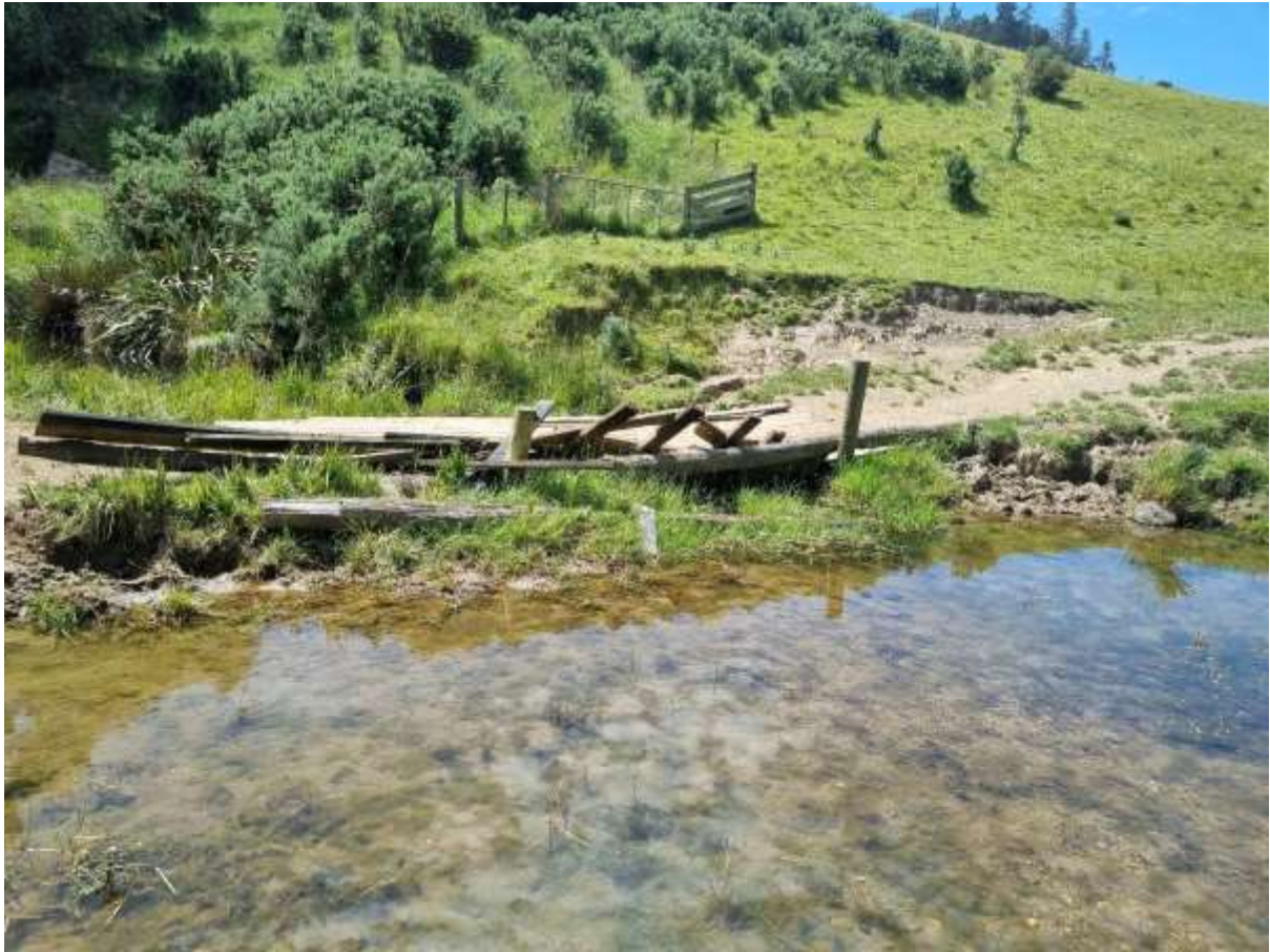
Figure 60 Downstream view of the H7 ford and bridge
