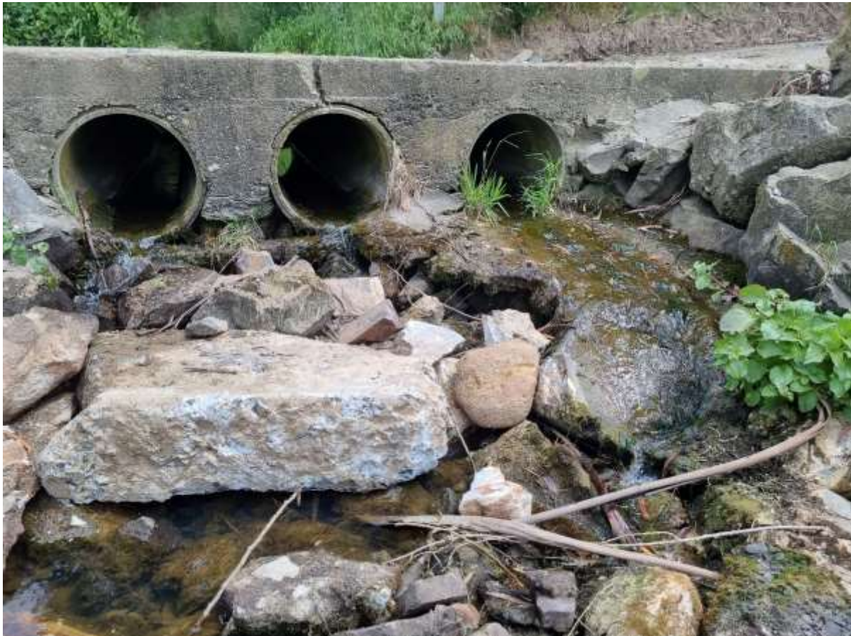
Figure 41 Downstream view of the H1 culverted ford
