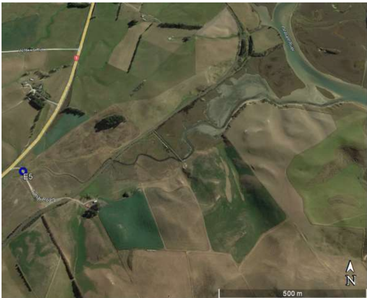
Figure 25 Location of the E5 culvert
