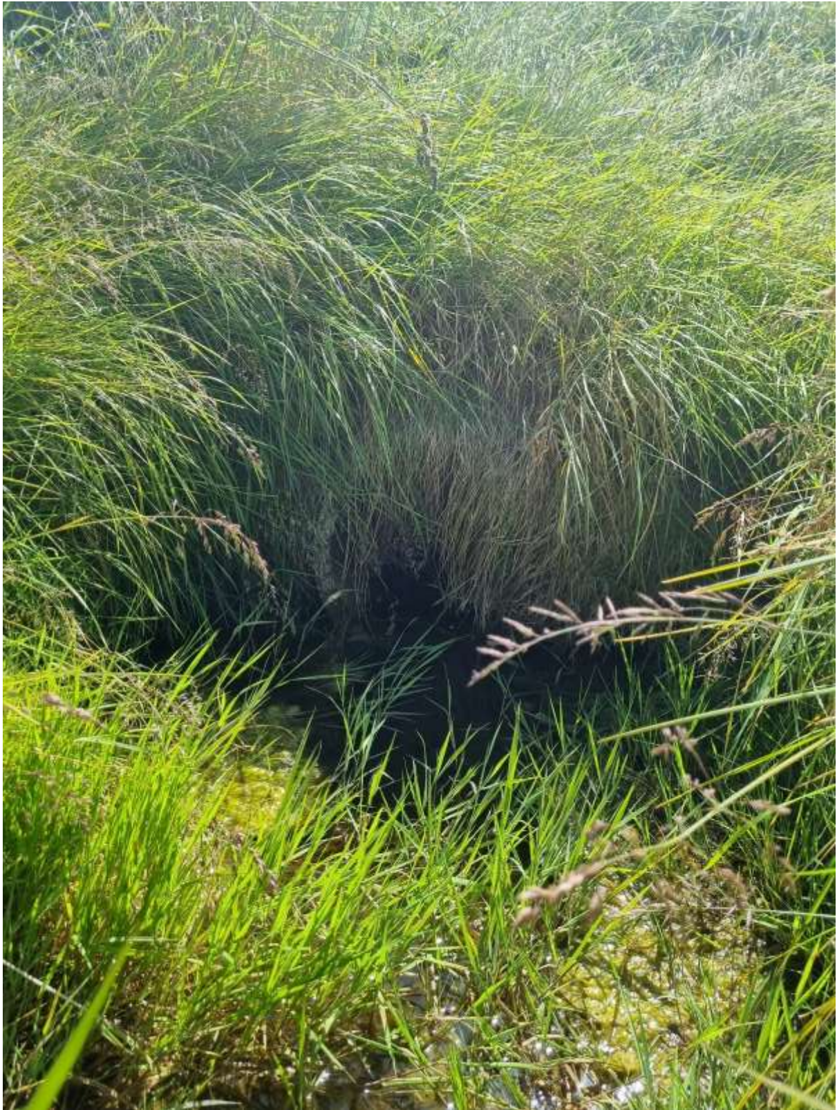
Figure 19 Upstream view of the E2 culvert
