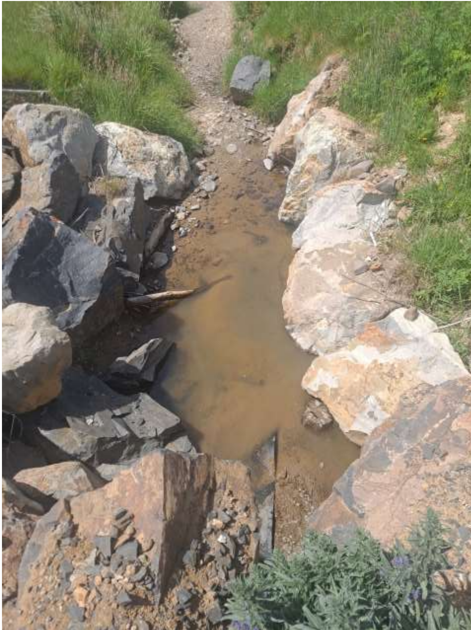
Figure 63 Downstream view from the H8 Culvert
