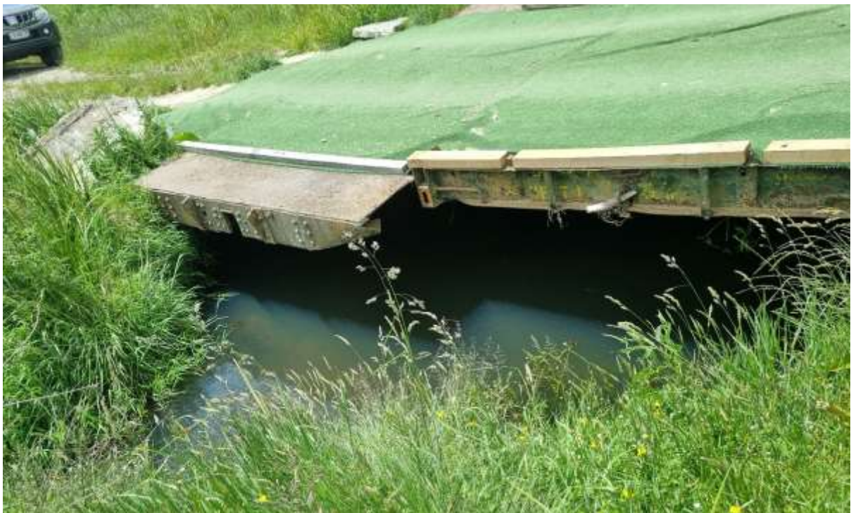
Figure 54 Downstream view of the H5 bridge
