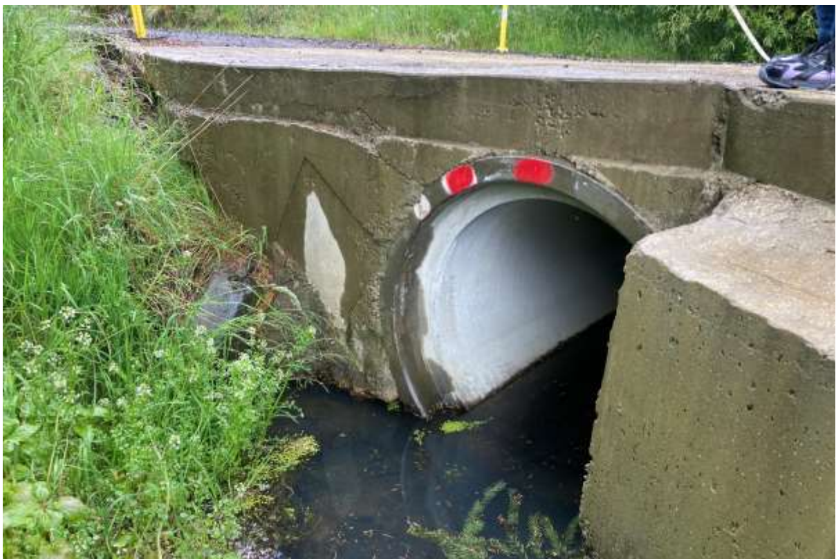
Figure 70 Upstream view of the H10 culvert
