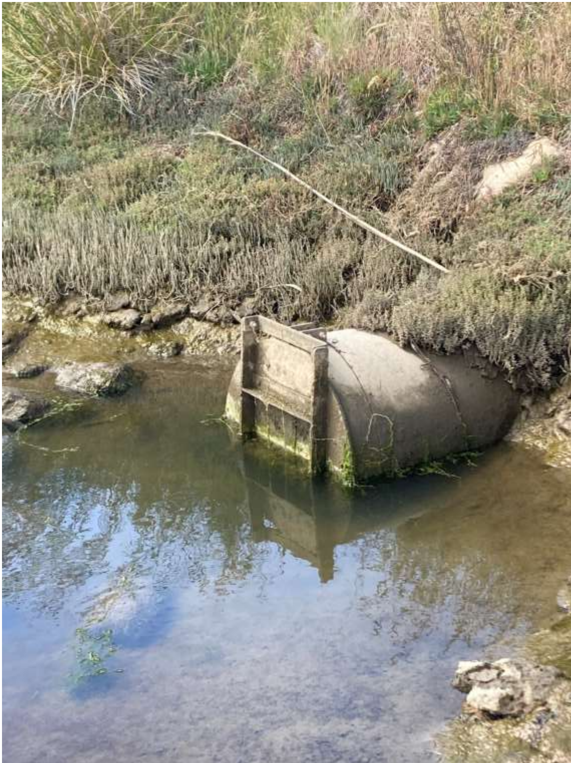
Figure 15 Downstream view of the E1 culvert
