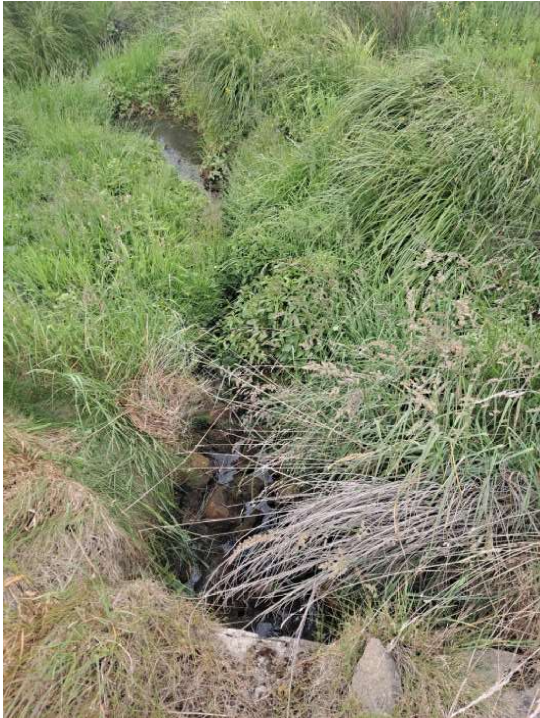
Figure 35 Downstream view from W3 culvert
