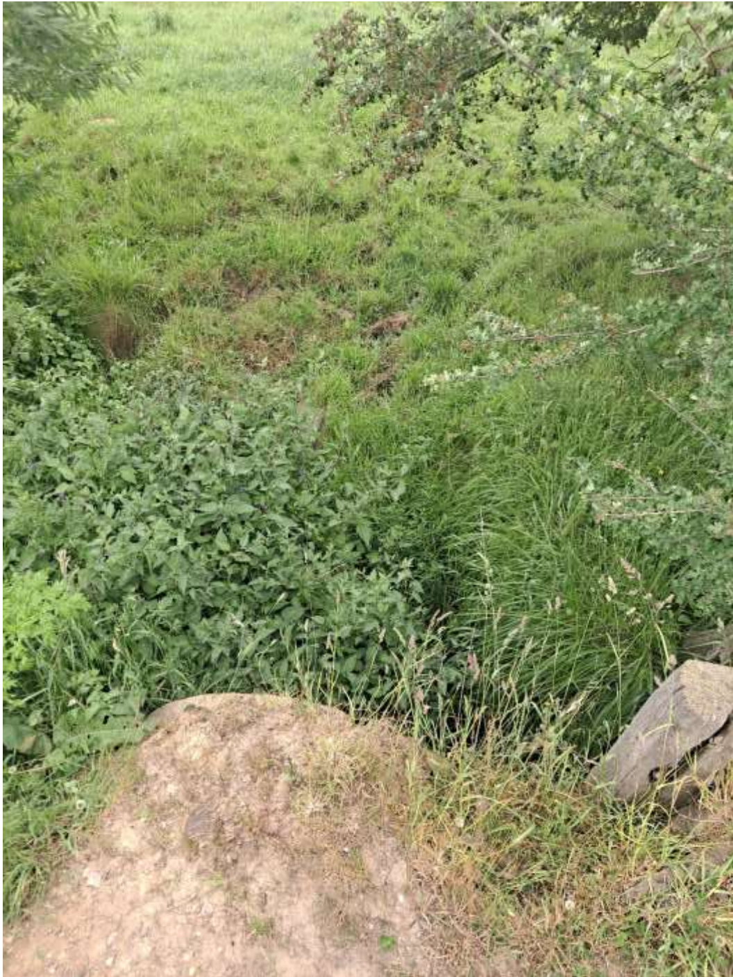
Figure 36 Upstream view from W3 culvert
