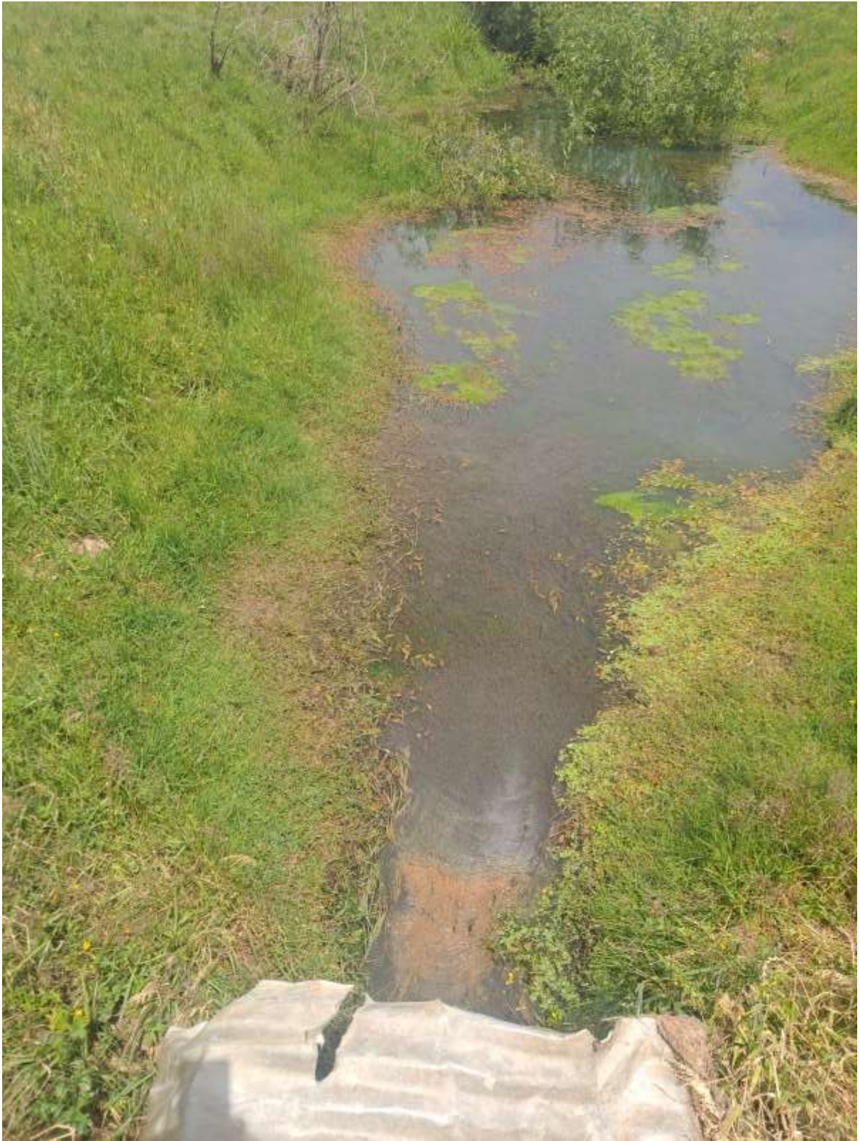
Figure 33 Upstream view from W2 culvert
