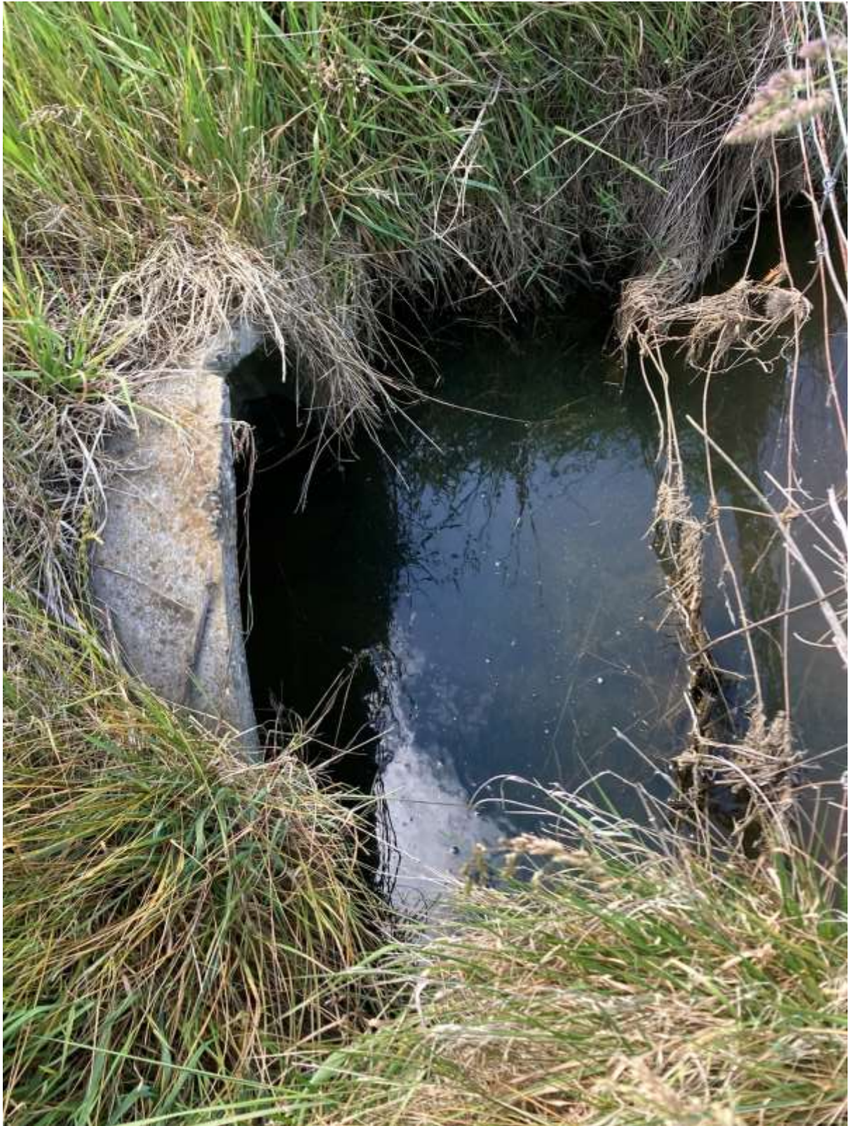
Figure 16 Upstream view of the E1 culvert
