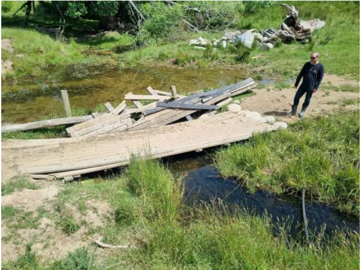
Figure 61 Upstream view of the H7 ford and bridge
