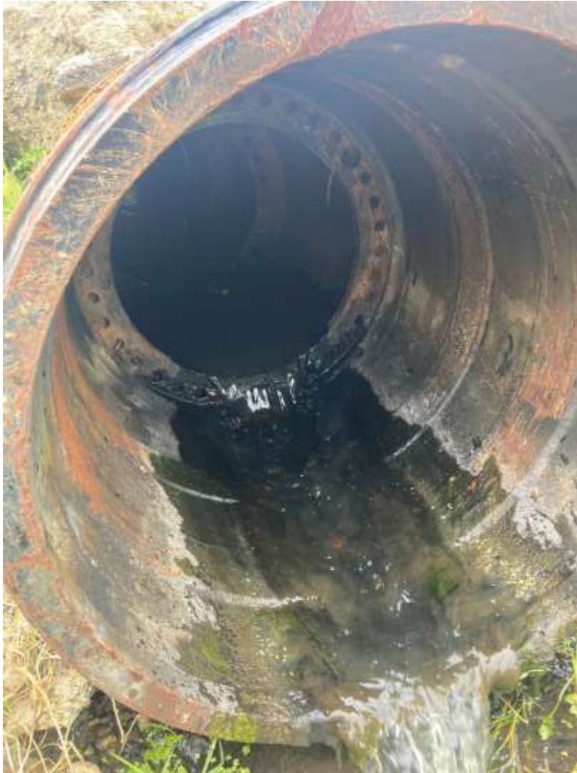
Figure 56 Internal view of the H6 culvert.
