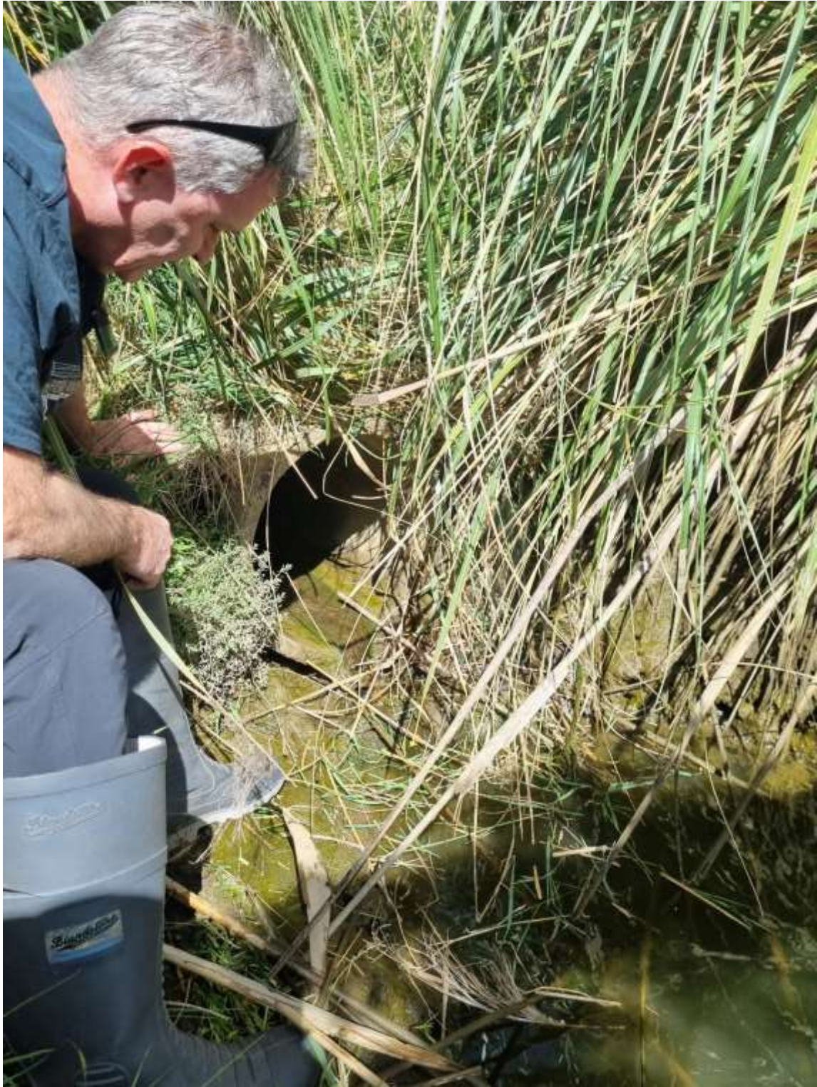
Figure 18 Downstream view of the E2 culvert
