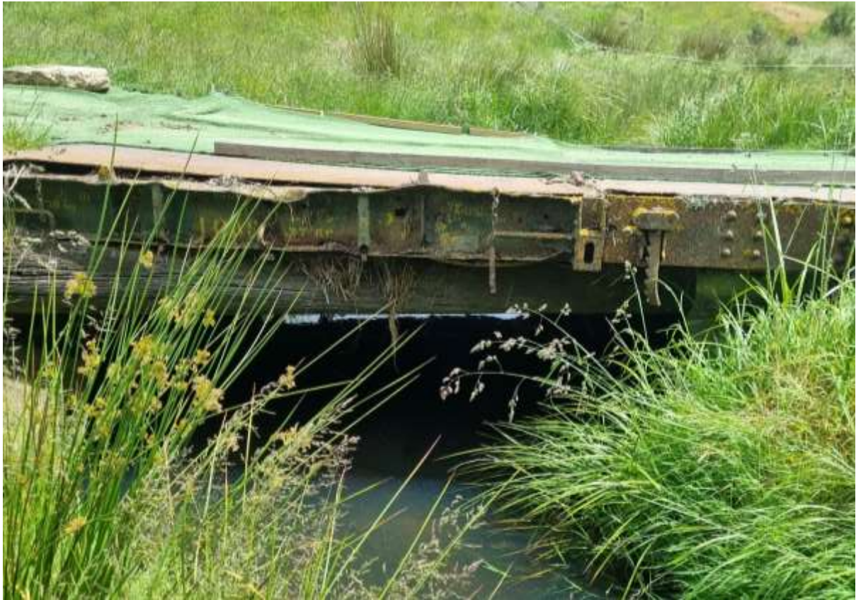
Figure 53 Upstream view of the H5 bridge
