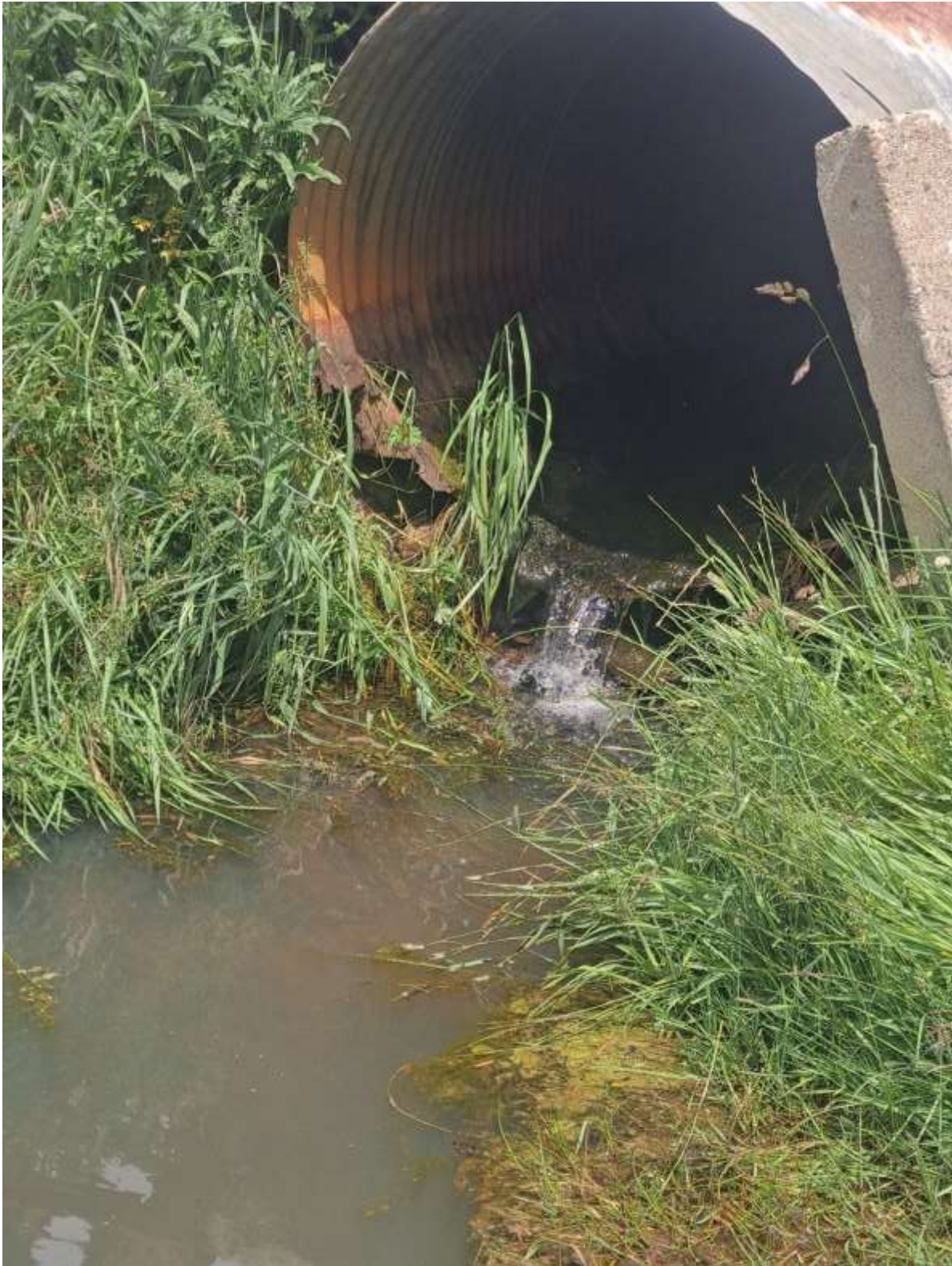
Figure 32 Downstream view of W2 culvert
