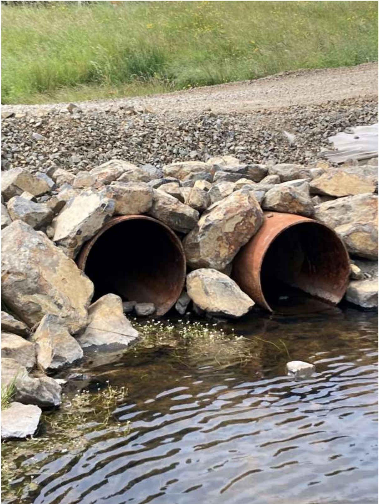
Figure 46 Upstream view of H2 culverts on December 13 th 2023
