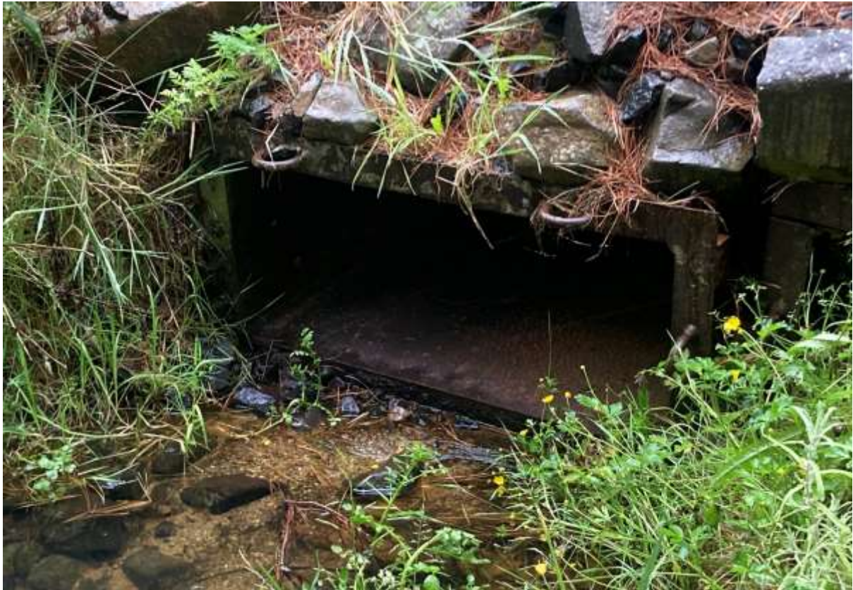
Figure 73 Upstream view of the H11 culvert
