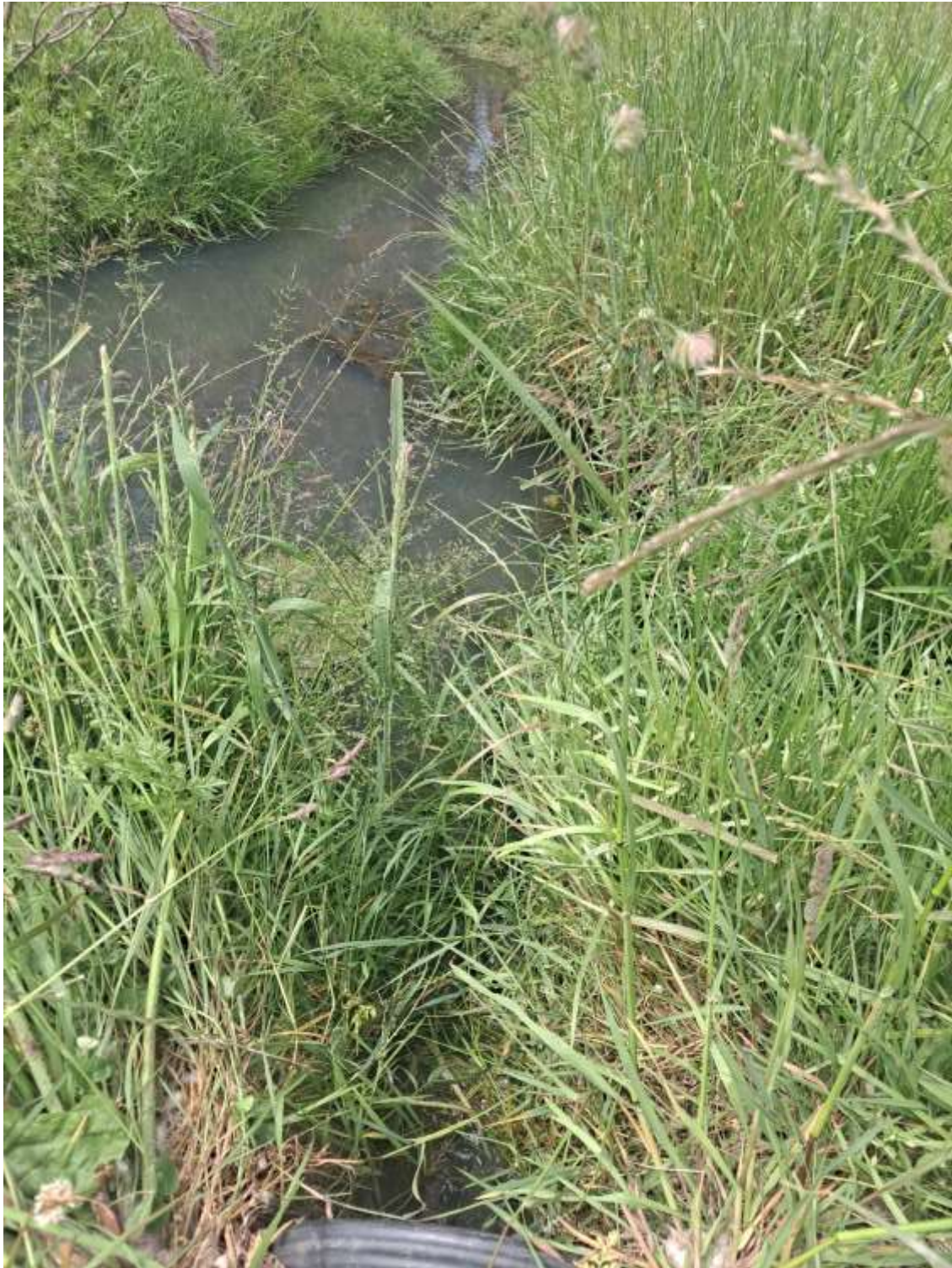
Figure 29 Downstream view from W1 culvert
