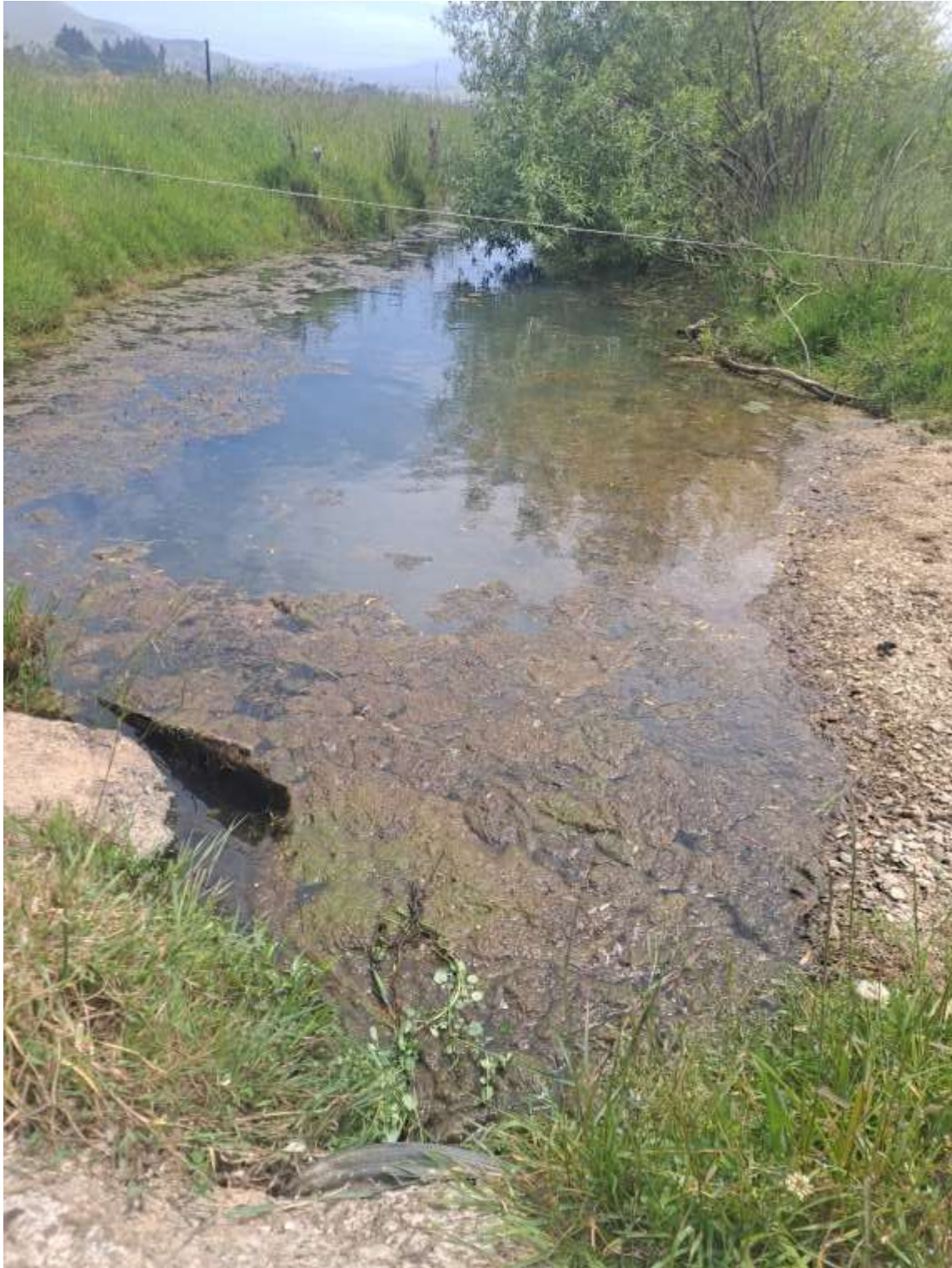
Figure 30 Upstream view from W1 culvert
