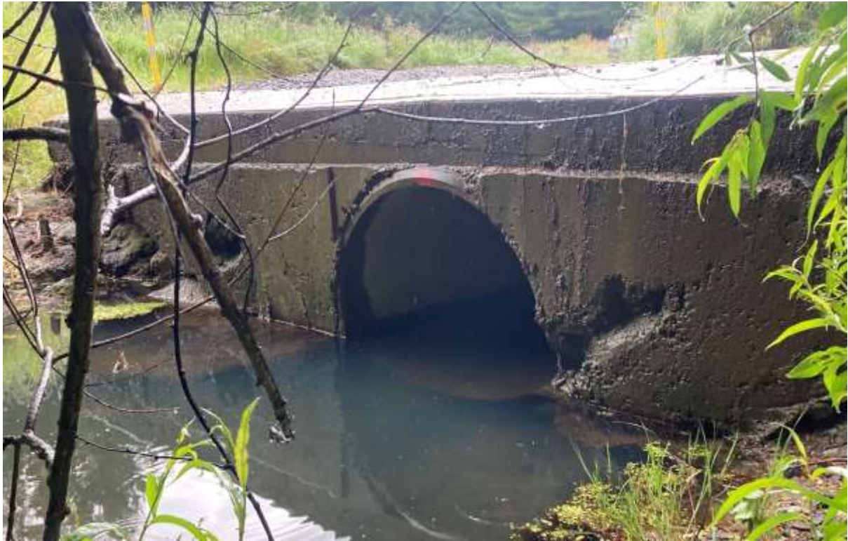
Figure 69 Downstream view of the H10 culvert
