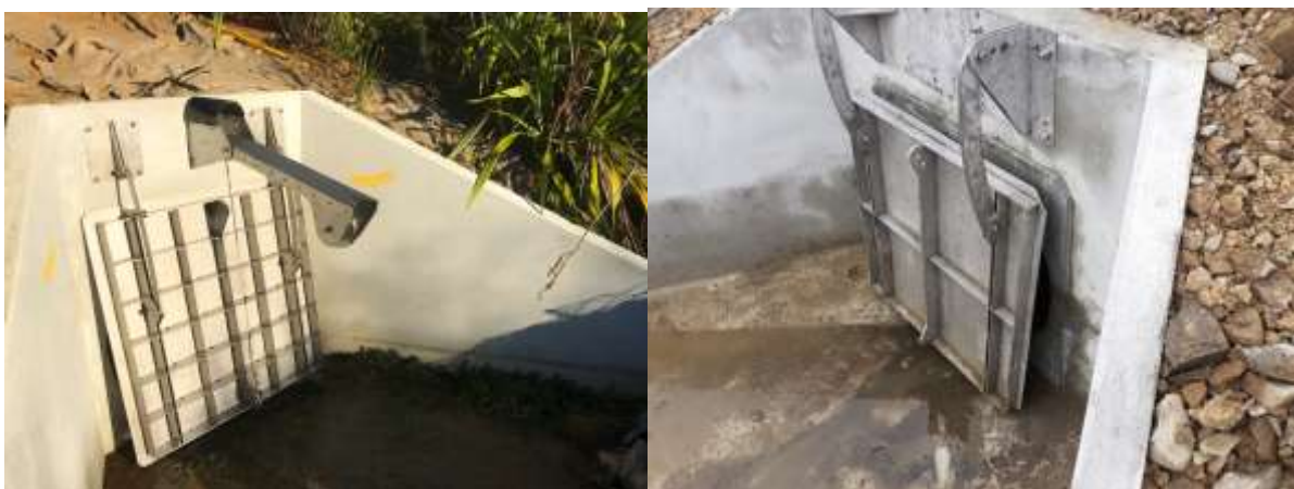
Figure 8 Examples of “fish friendly” flap gates. The cantilever gate on the left, and the offset top hinged on the right.
