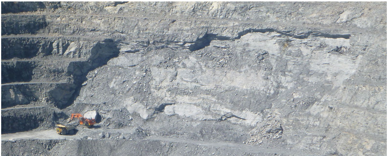
Photo 3: Frasers east wall failure during mining showing the interim base of failure at 330 mRL.
