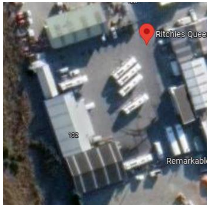
Figure 53: Existing Ritchie's bus depot on Glenda Drive, Frankton
