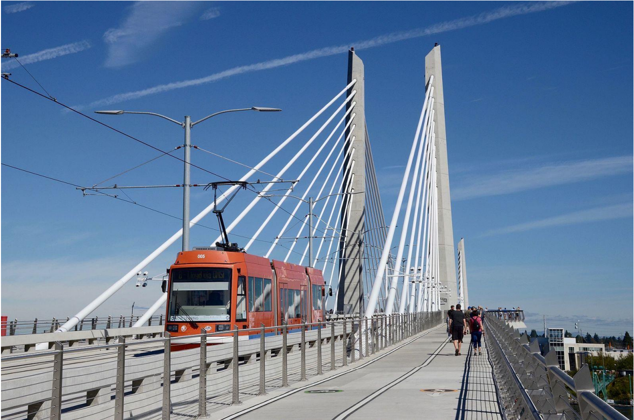
Figure 43. Example of public transport, cycling and walking only bridge, Tilikum Crossing Portland (Source: Archdaily).
