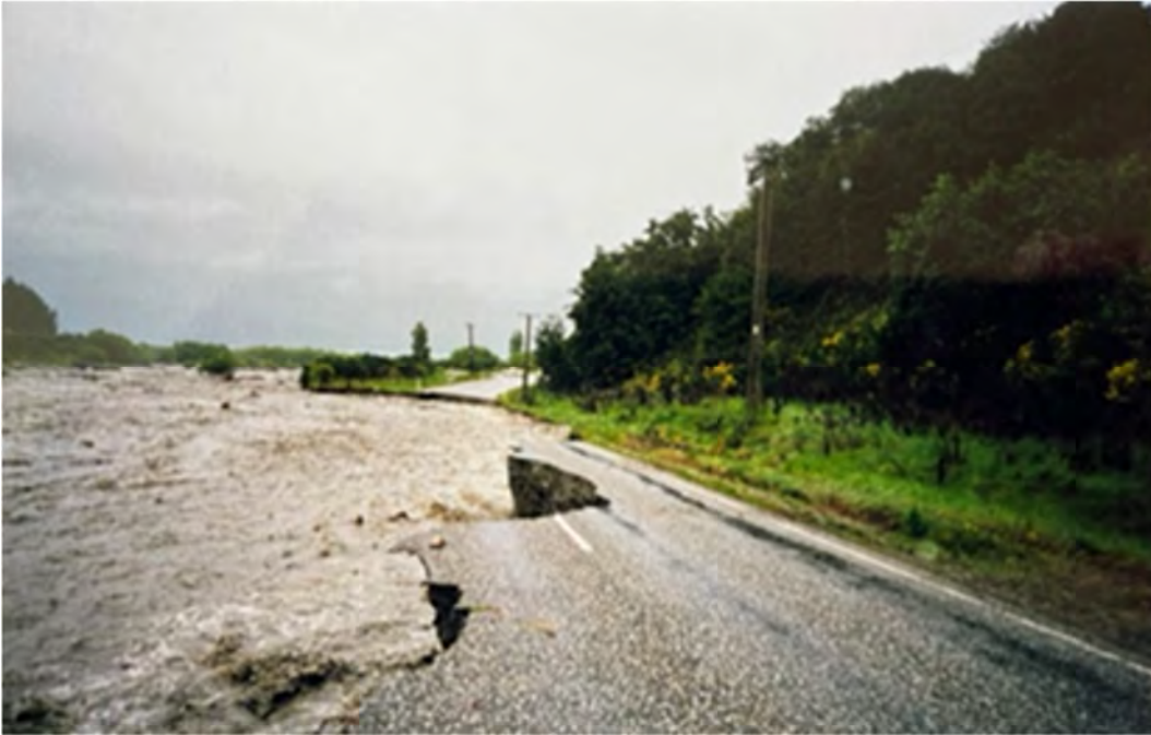
Figure 2-5: Glenorchy - Queenstown Road is washed out by Buckler Burn during the 1999 flood event. Photo credit: Kelly Family.
