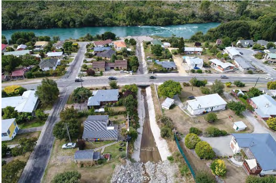
Figure 7: The Reservoir Creek concrete chute, constructed in the early 1980s.
