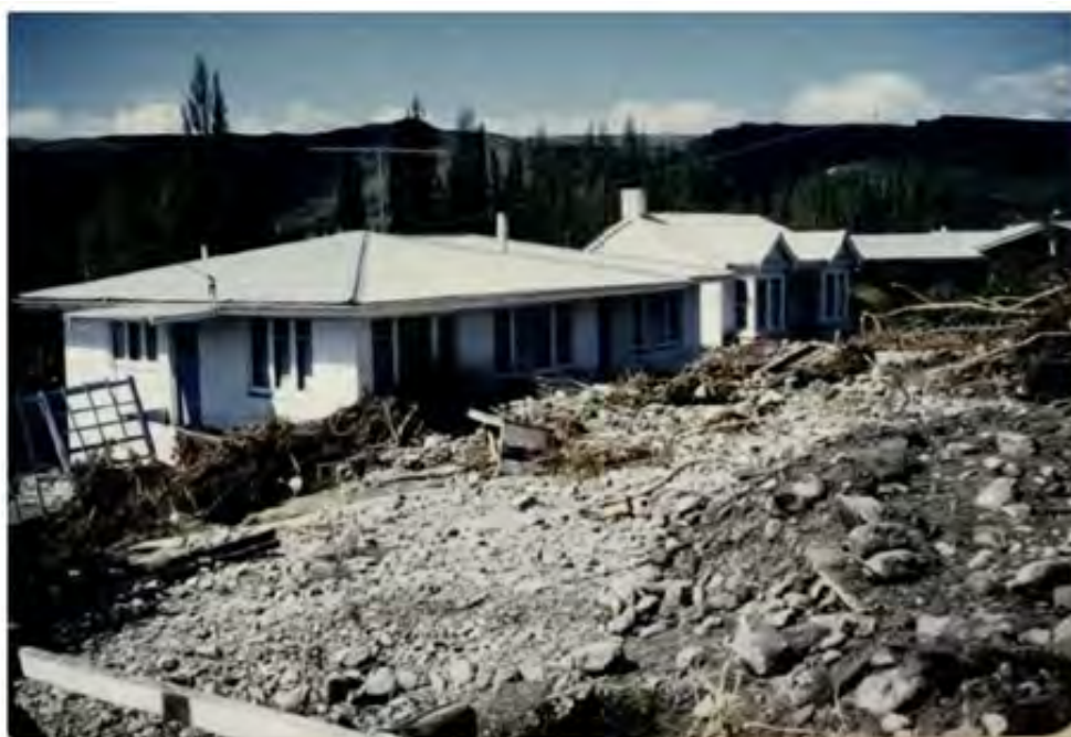
Figure 6: Direct impact of a debris flow at Reservoir Creek, 1978, showing extensive debris deposition, and direct impact to dwellings adjacent to the stream channel.
