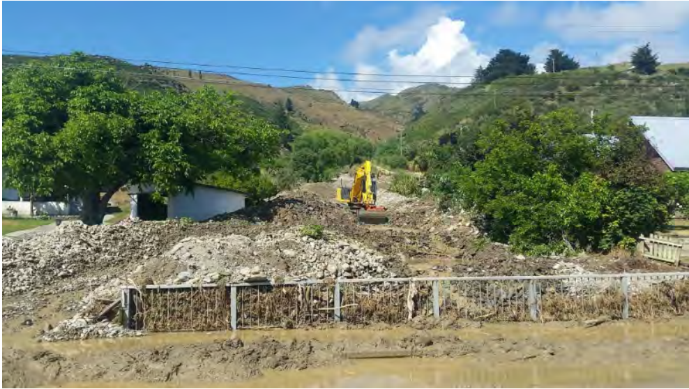
Figure 9: Impacts of the November 2017 events at Reservoir Creek, looking upstream of the SH8 bridge.
