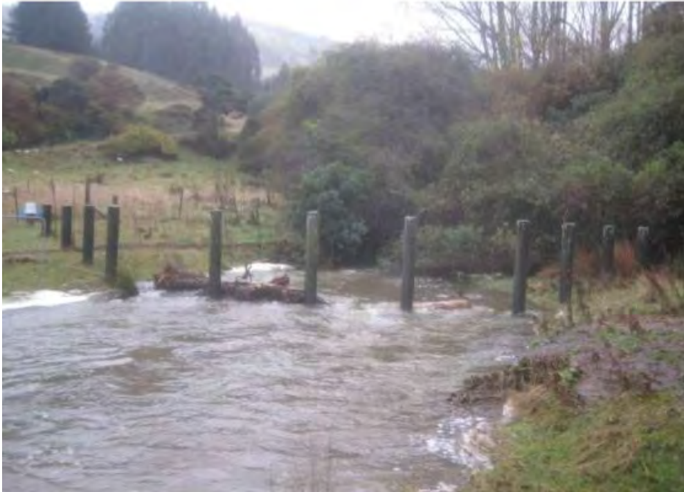
Figure 8. Lindsay Creek debris trap (looking upstream), 3 June 2015. The peak flow in this event was ~30 cumecs (measured at North Road Bridge), however the photo is not necessarily showing the period of peak flows.
