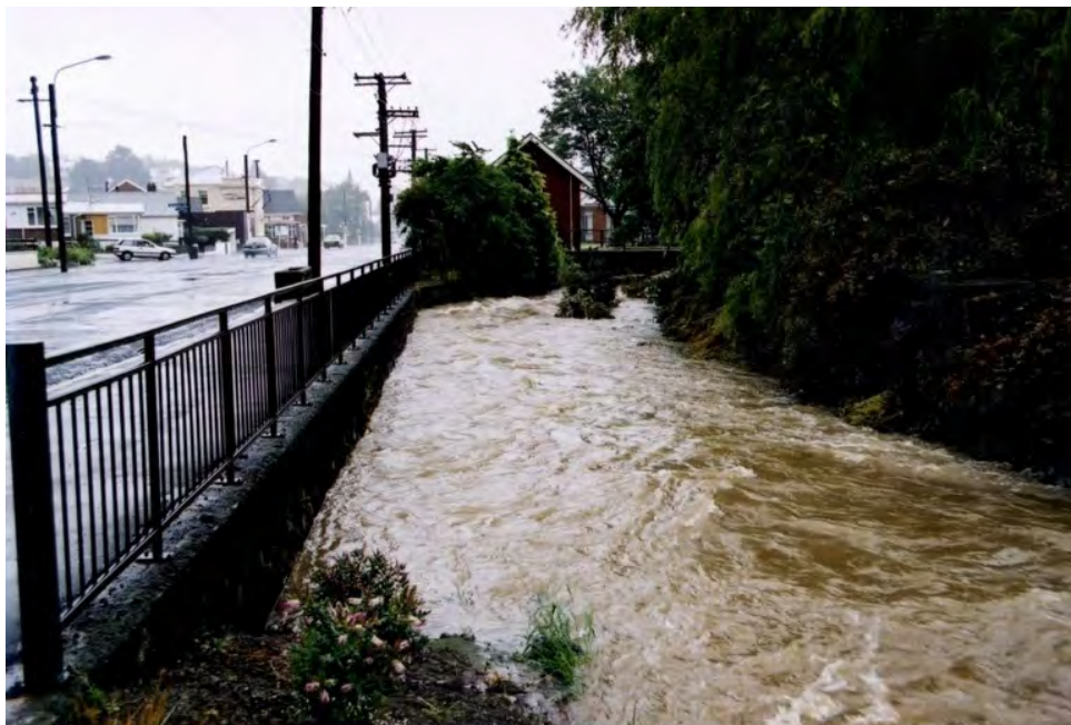
Figure 4. View downstream on Lindsay Creek at Palmers Quarry Bridge during a January 2002 flood event (12 January 2002). Note the very limited freeboard remaining until floodwaters would overtop the left bank onto North Road. The peak flow in this 2002 event was \sim 19 \text{ m}^3/\text{s} , well below peak flows of 30\text{-}32 \text{ m}^3/\text{s} recorded in 1991, 2006 and 2015. Photograph is not necessarily taken at the peak of the high flows for the event.
