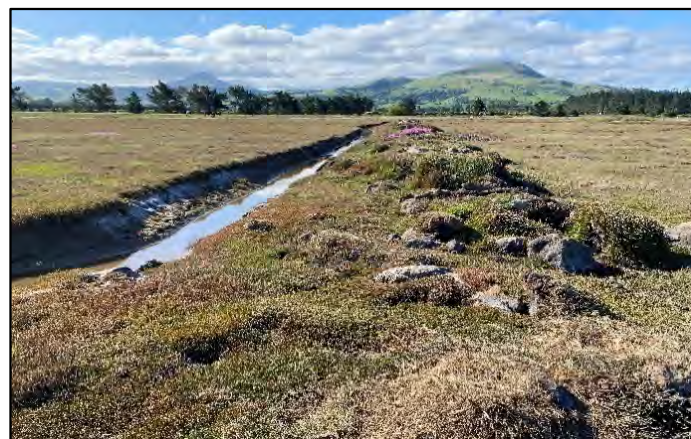
New drainage channels dug out of the salt marsh post-2020.
