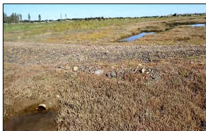
Small causeway installed across a channel of East Arm.
