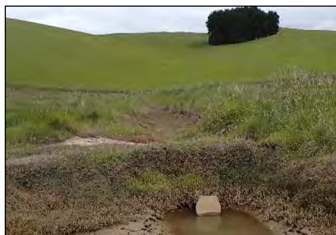
Flap gate preventing tidal inundation into low lying paddock.
