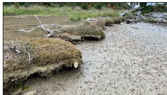
Erosion on the margin of the upper estuary channel.
