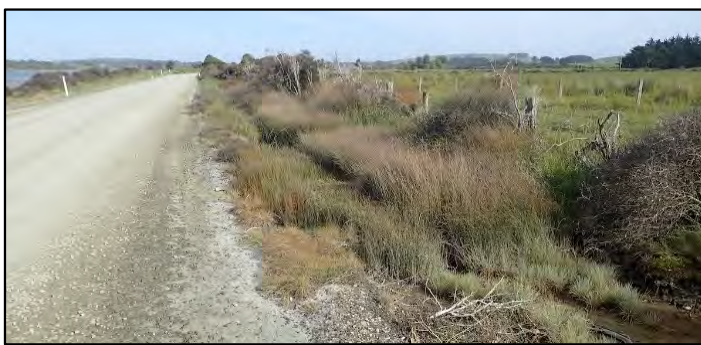
Tidal drainage channels with salt marsh species on the landward side of the road edge.
