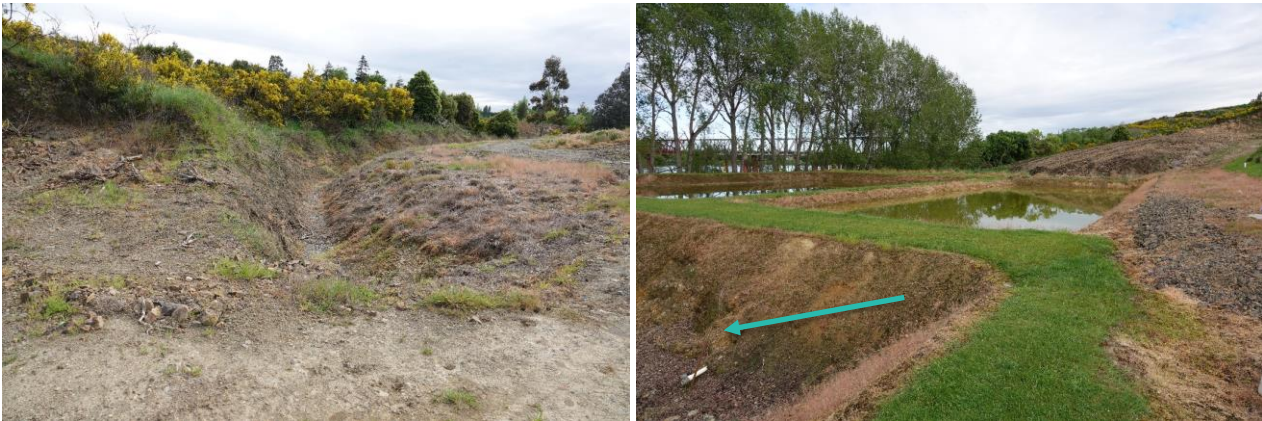
Figure 5: Stormwater diversion drain (left) and detention pond overflow drain (right, arrowed).
