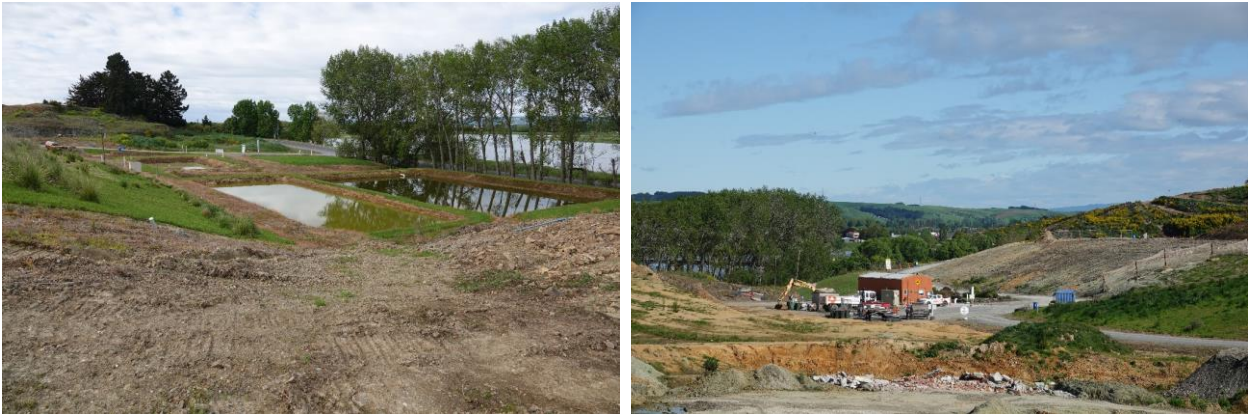
Figure 2: Stormwater retention ponds and plantings (left), and buildings and roads (right).
