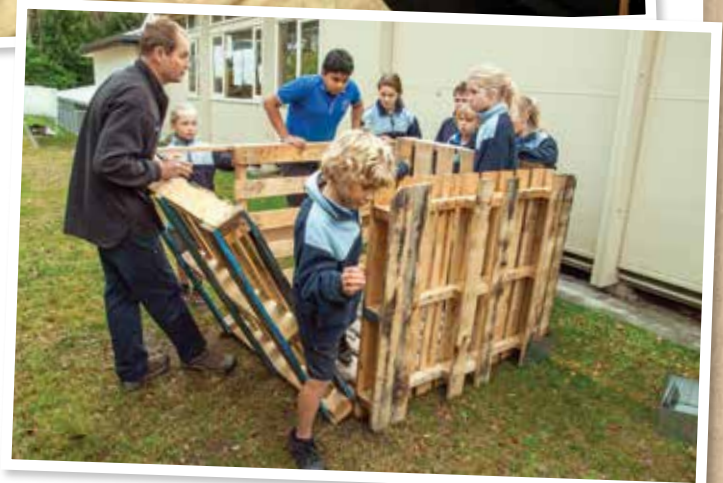
Building the Compost Bins
