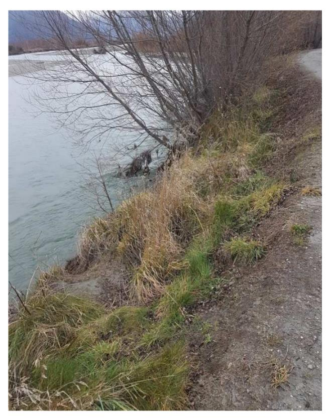
Site 6 - Rees river running against the base of the flood bank, undermining the bank
