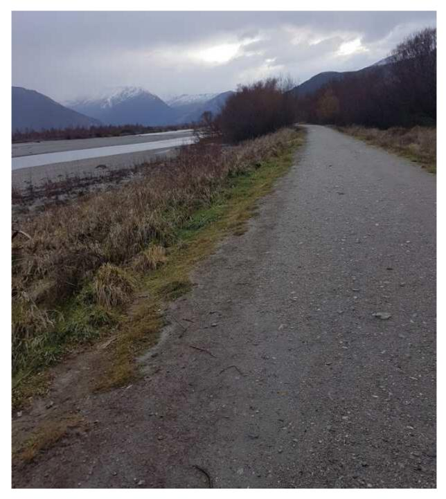
Site 11 - General section of trail with a drop in trail level and the formation of a headscarp on the water side.
