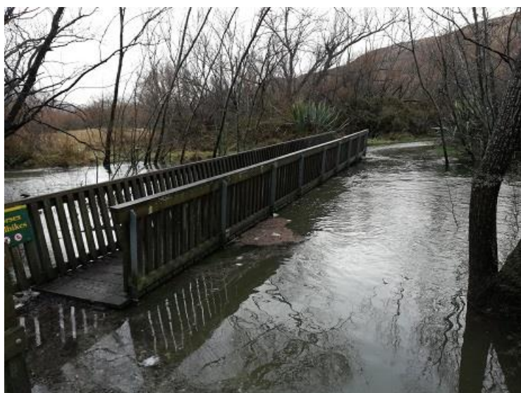
Figure 1 - Lagoon Bridge 21st June. Photograph Ingrid Temple to Ulrich Glaser
