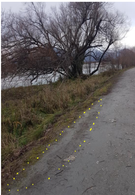
Figure 7 - Indicative surface slumping of the embankment crest
