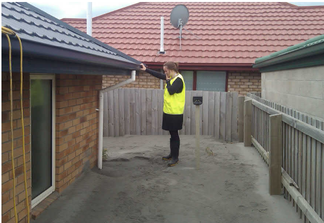
Figure 10.10 Inundation from ejection of sand from liquefaction, Christchurch 2010
