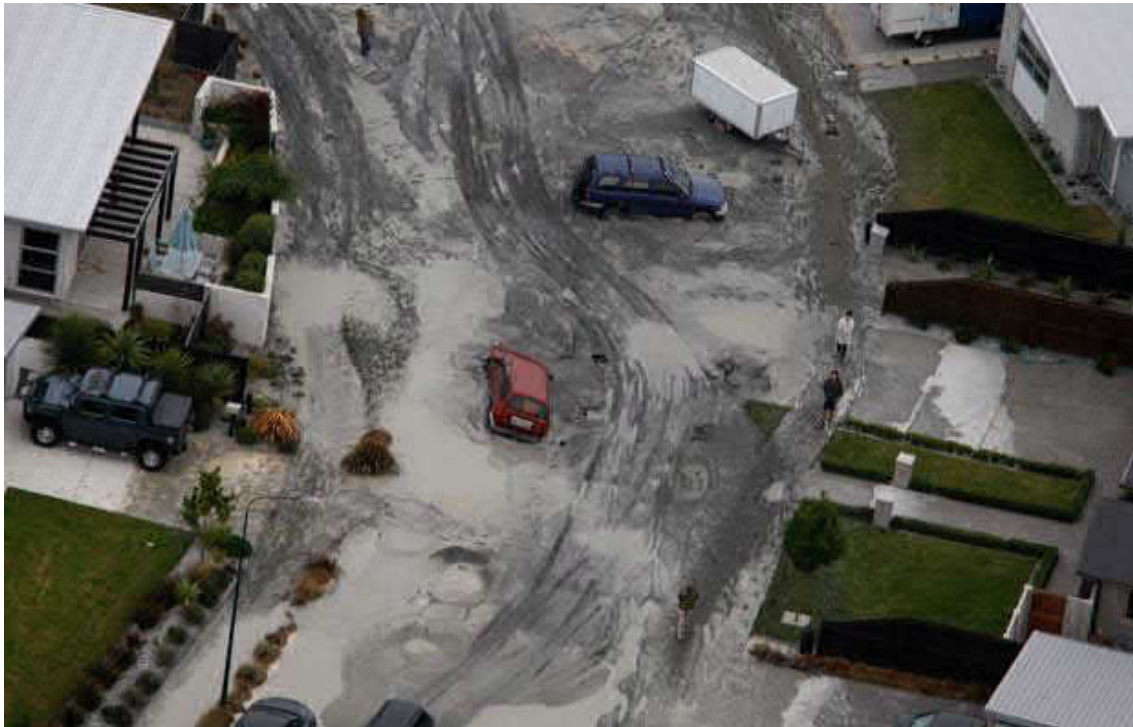
Figure 10.8 Inundation from ejected sand and water from liquefaction, Christchurch 2011 (EQC)
