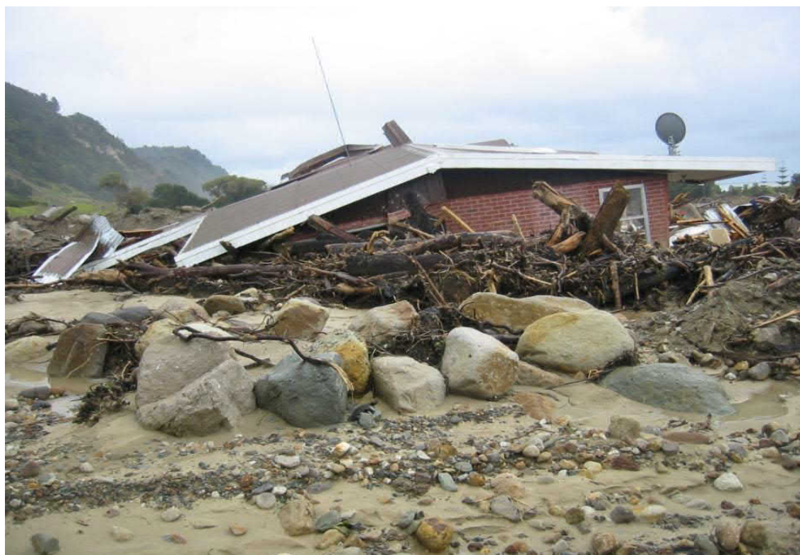
Figure 10.2 Rainfall triggered debris flow (Matata 2005)
