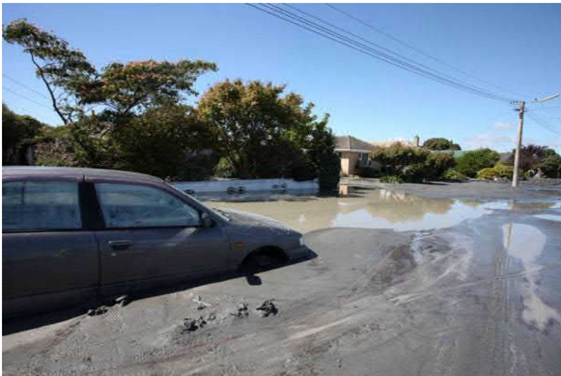
Figure 10.9 Inundation from ejected sand and water from liquefaction, Christchurch 2011
