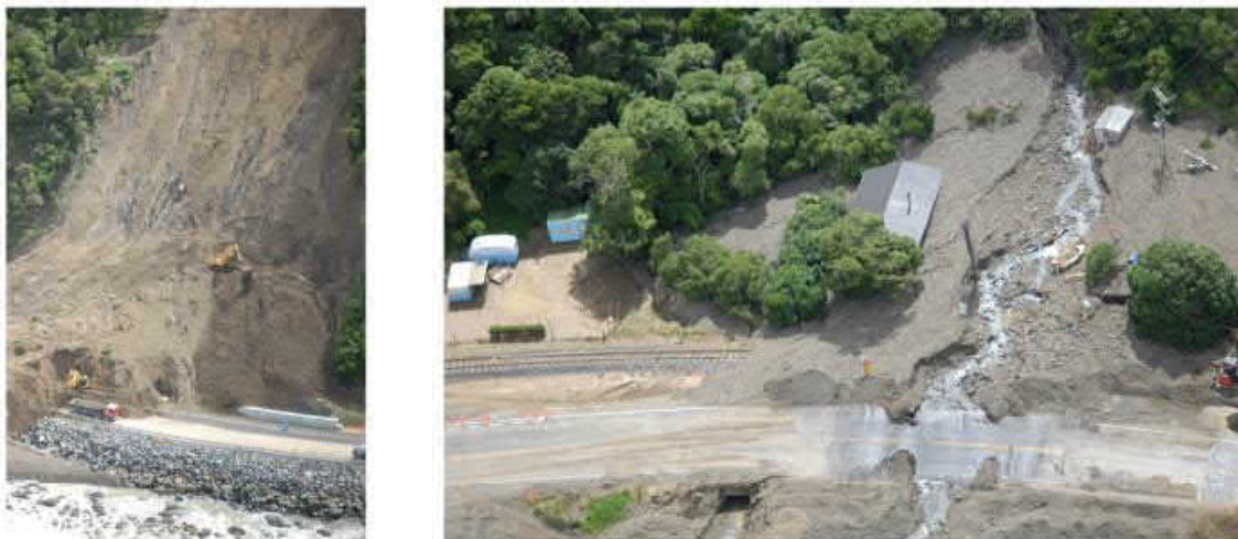
Figure 10.6 Rainfall induced debris flows 2018 post Kaikoura Earthquake 2016 (GNS Science) Note the size of the debris protection wall relative to the size of the debris flow, in the left image
