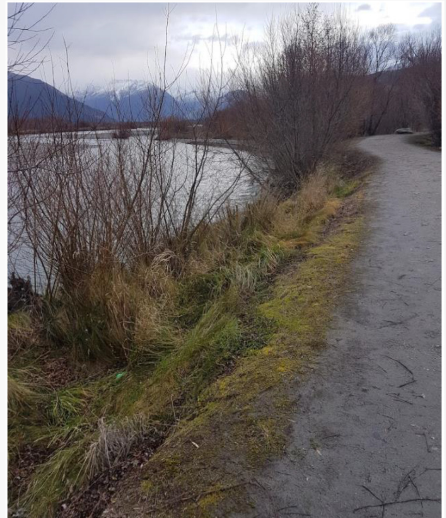
Headscarps forming at over steep bank downstream of the Lagoon stream confluence
