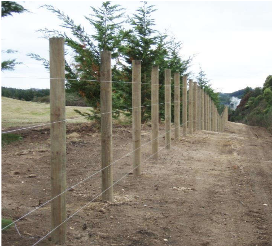
Figure 1-3: Section of base fence prior to installation of pest-proof components.
