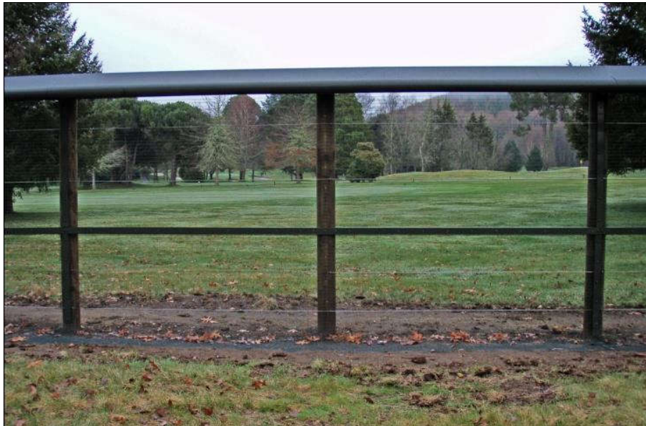
Figure 3: Panel view of Xcluder® “All-Pest” fence.
