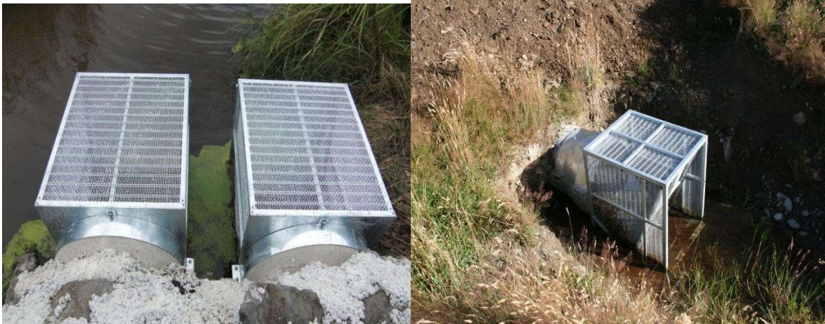
Figure 1-1: Galvanised mesh culvert cubes to provide pest-proofing on water table pipes.
