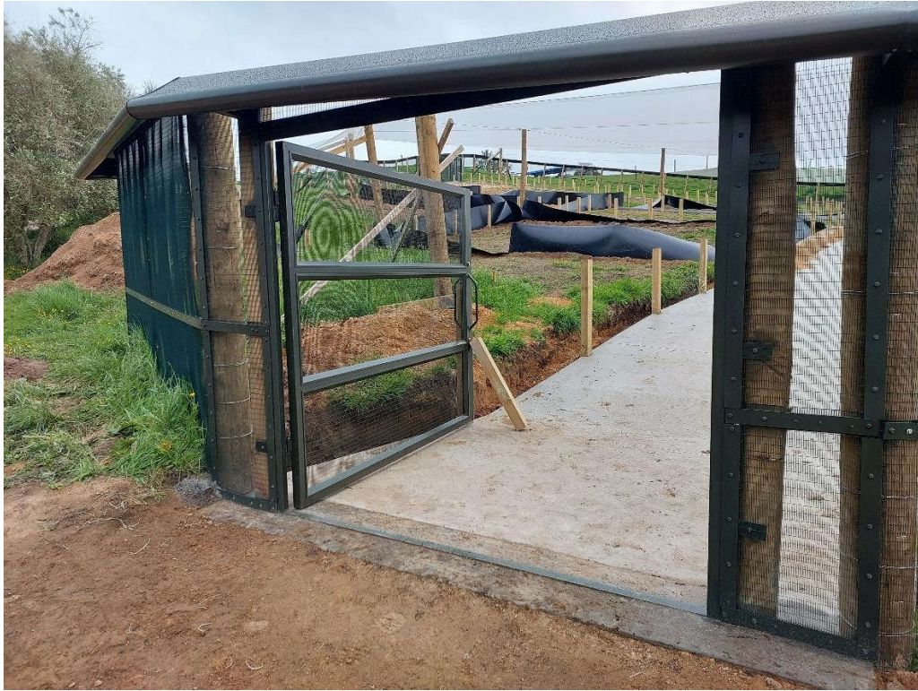
Figure 1-7: Xcluder® self-shutting ATV access gate under construction at the Agrodome.
