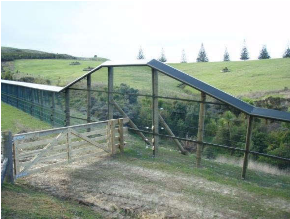
Figure 1-4: Xcluder® "up-and-over" structure for an abutting fence.
