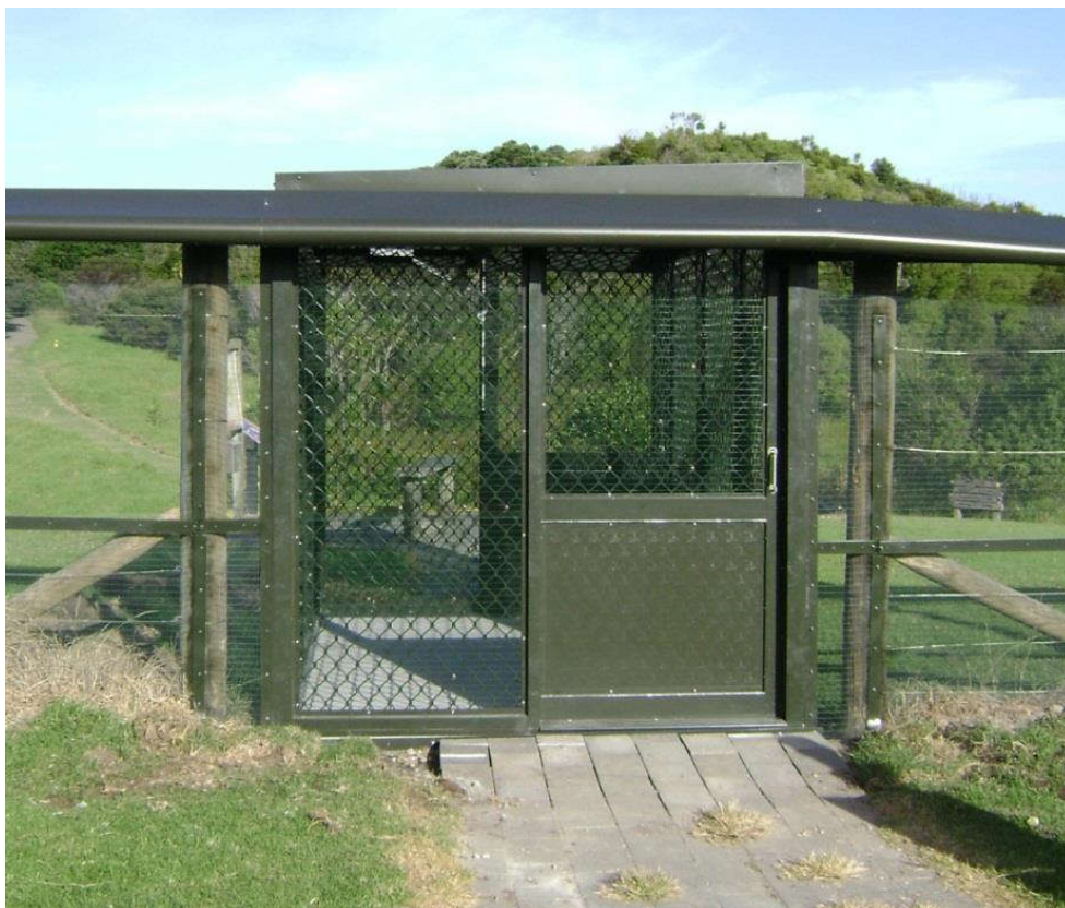
Figure 1-6: Xcluder® pedestrian access gate at Shakespear Peninsula, featuring interlocked, self-shutting sliding doors in a 3 × 2 metres aluminium cage.
