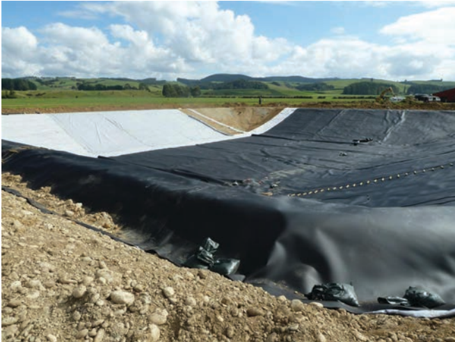
Geomembrane with geotextile underliner being installed.
