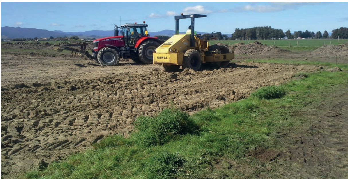
Trial Compaction Area Preparation
