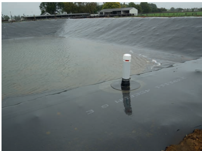
Lining with gas vent.
