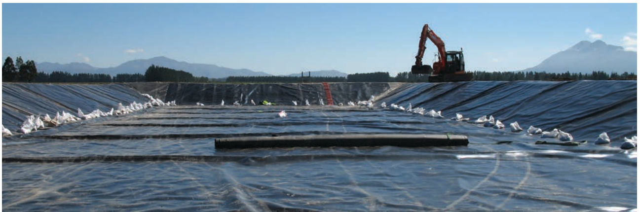
HDPE synthetic liner being installed
