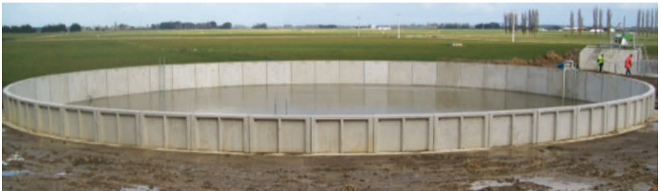
2,000m 3 precast concrete tank
