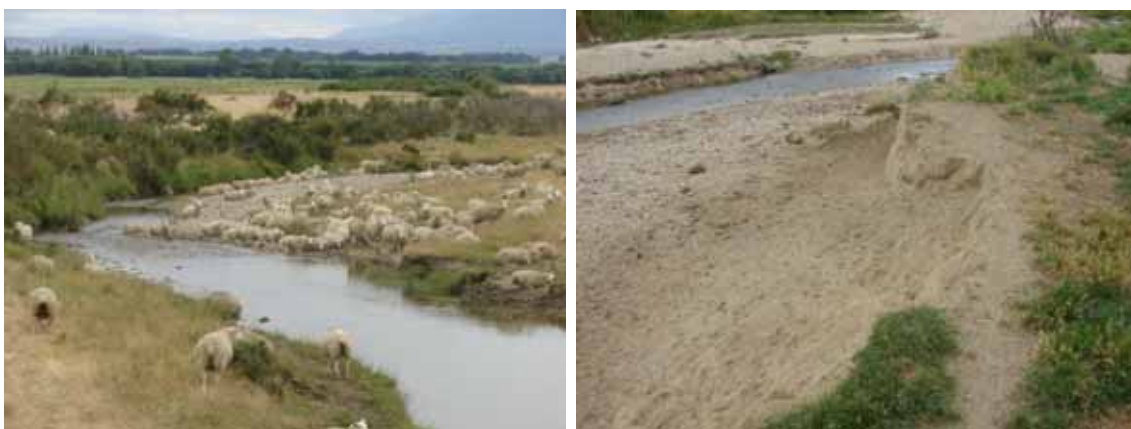
Figure 5.2 Unrestricted stock access in Sow Burn allows stock to erode the banks which then act as a sediment source when flows increase.
