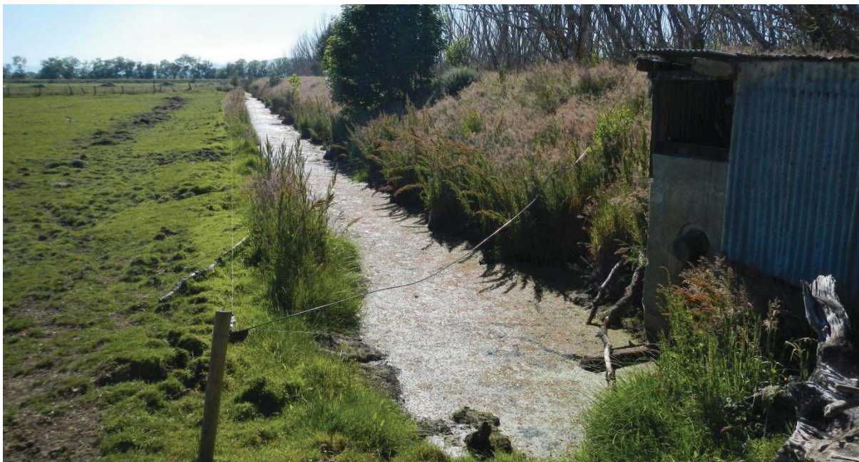
Figure 2: The floodbank, drain and pumpstation that separate the pastureland on the Beaton property from the Waipori/Waihola Wetlands Complex.
