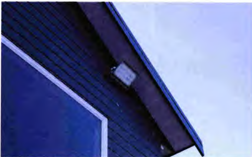
Figure 6 Symmetrical LED floodlight at wharf
