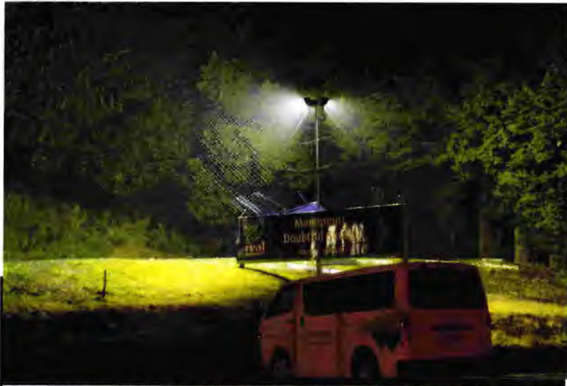
Figure 14 Floodlighting in staff car park with upward light component visible
