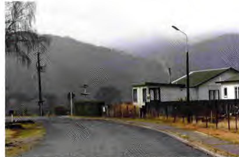
Figure 17 Street lights in Monowai with 45° tilt angle creating significant upward light spill. Changing these HPS luminaires to LED without adjusting the tilt angle to 0° will impact on the night sky and potentially create a traffic hazard and glare issues for neighbours
