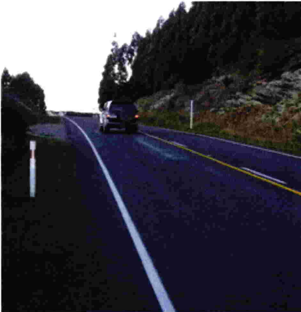
Figure 2: Milford Road immediately north of the Upukerora Bridge
