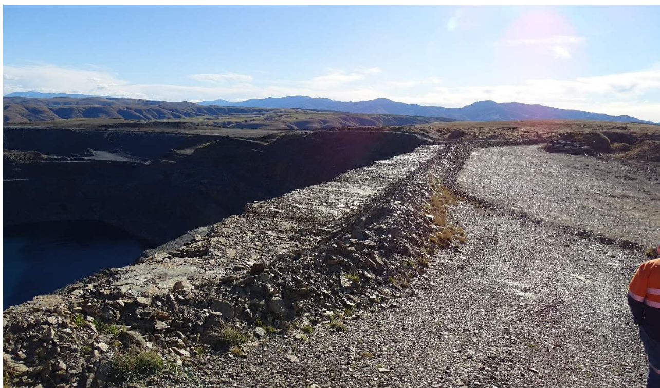
Figure 2-6. View of Coronation Pit from the southeast side looking to the north
