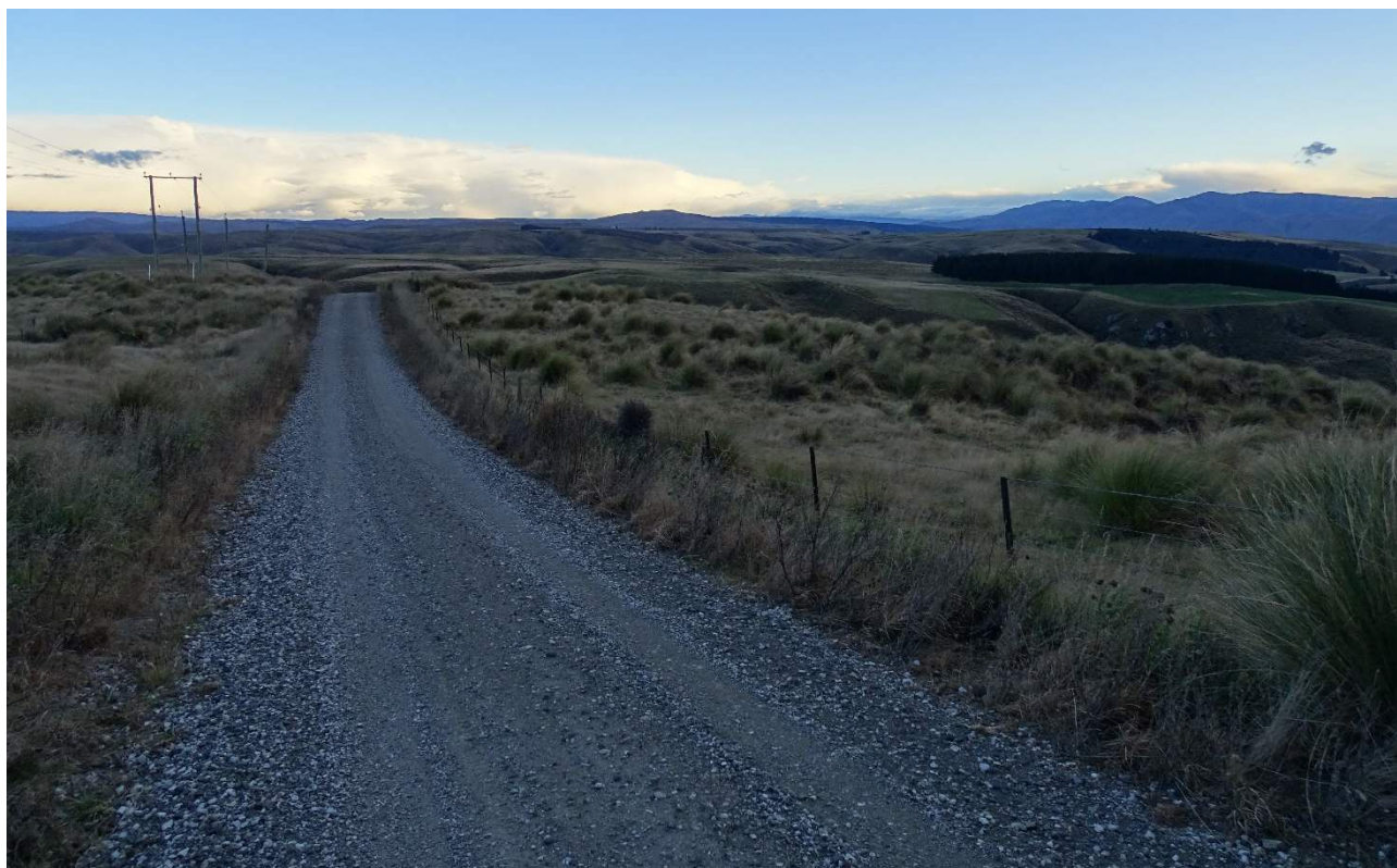
Figure 2-16. View towards Golden Bar Pit from the northwest side including Golden Bar Road
