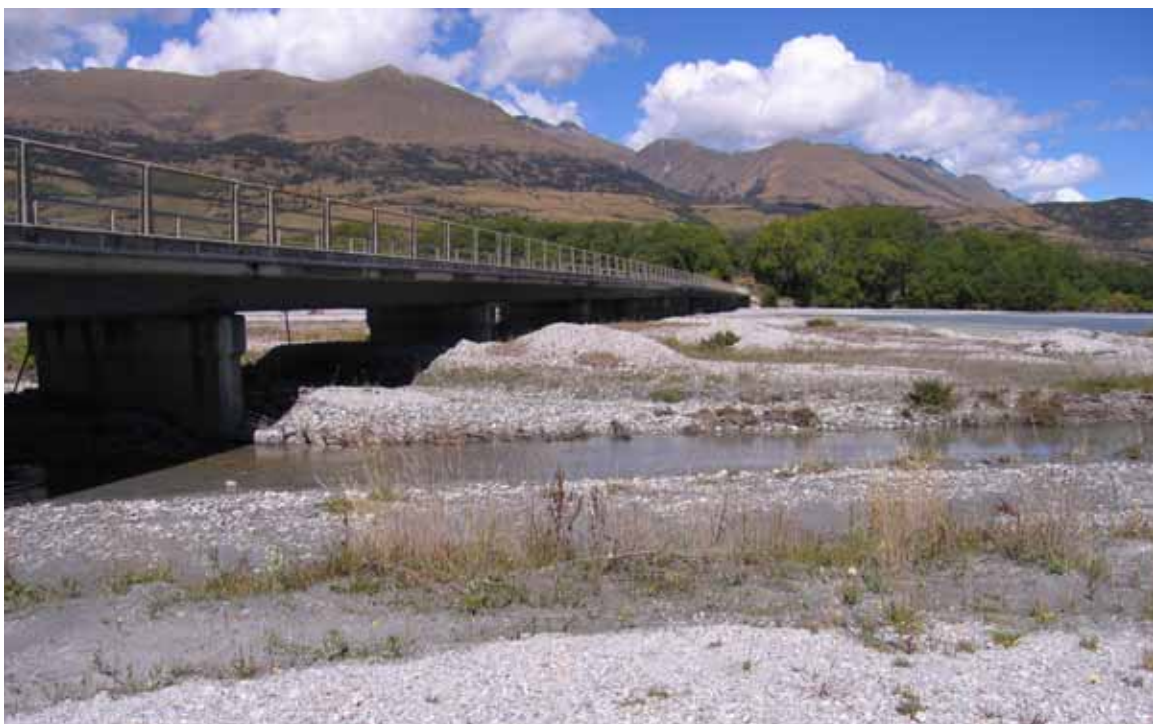
Figure 3.10 Photograph showing the Rees River bridge on the downstream side looking towards the true left, February 2008
