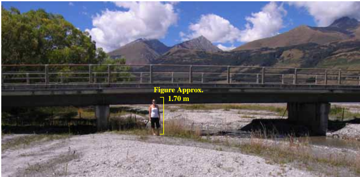
Figure 3.9 Photograph showing the Rees River bridge on the true right bank looking upstream, February 2008
