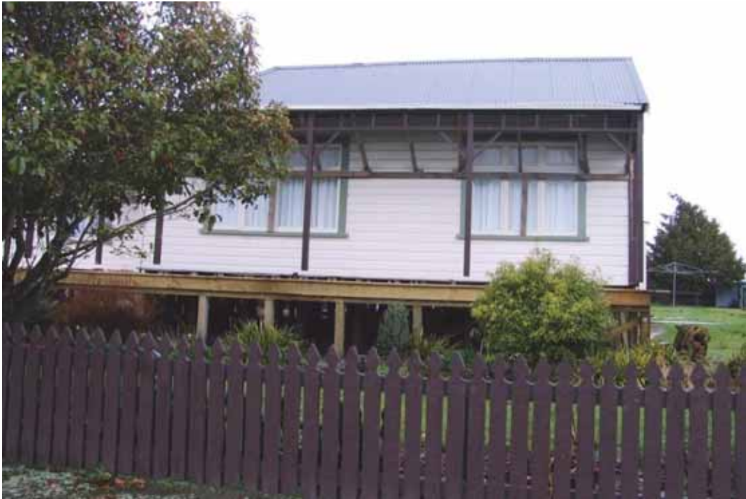
Figure 8. Residential building on raised foundations.
