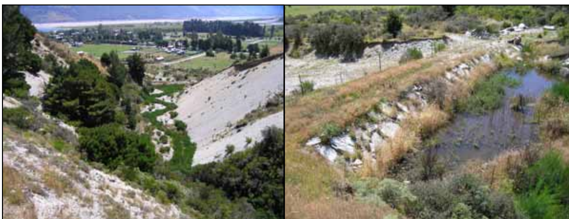
Figure 3.18 The Bible Stream Gully (left) and associated dam embankment (right)
