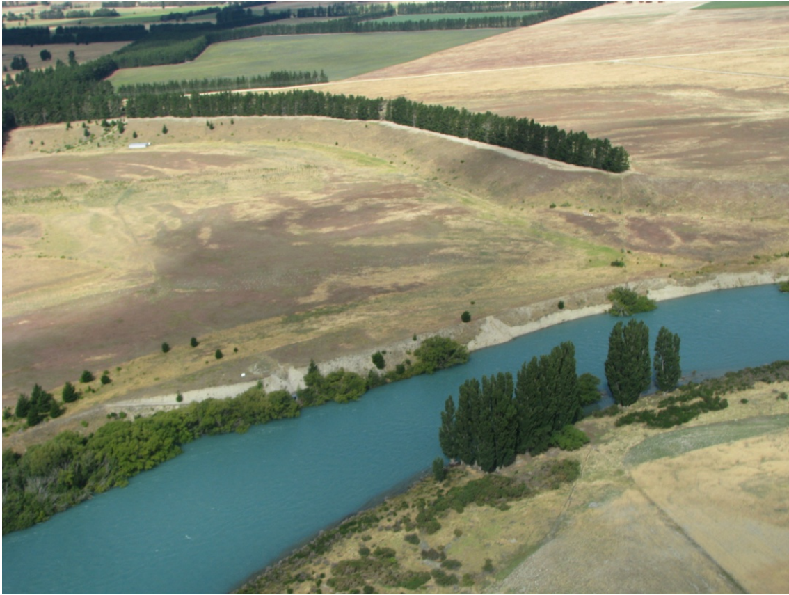
Figure 20. View of the Clutha River/Mata-Au, looking downstream and showing erosion of the true left bank, downstream of Queensberry (point 2 on Figure 15). Photo taken 15 January 2013.
