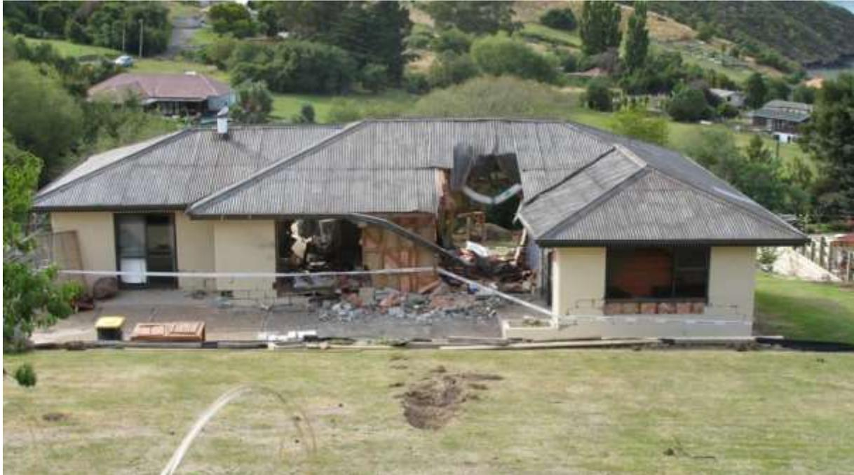
**Figure 8. Rockfall damage to dwelling at Rapaki, Christchurch, during Feb. 22nd 2011 earthquake. The gouge in the foreground is an impact divot from a boulder, which then impacted the house (photo courtesy D. Barrell, GNS Science).**
