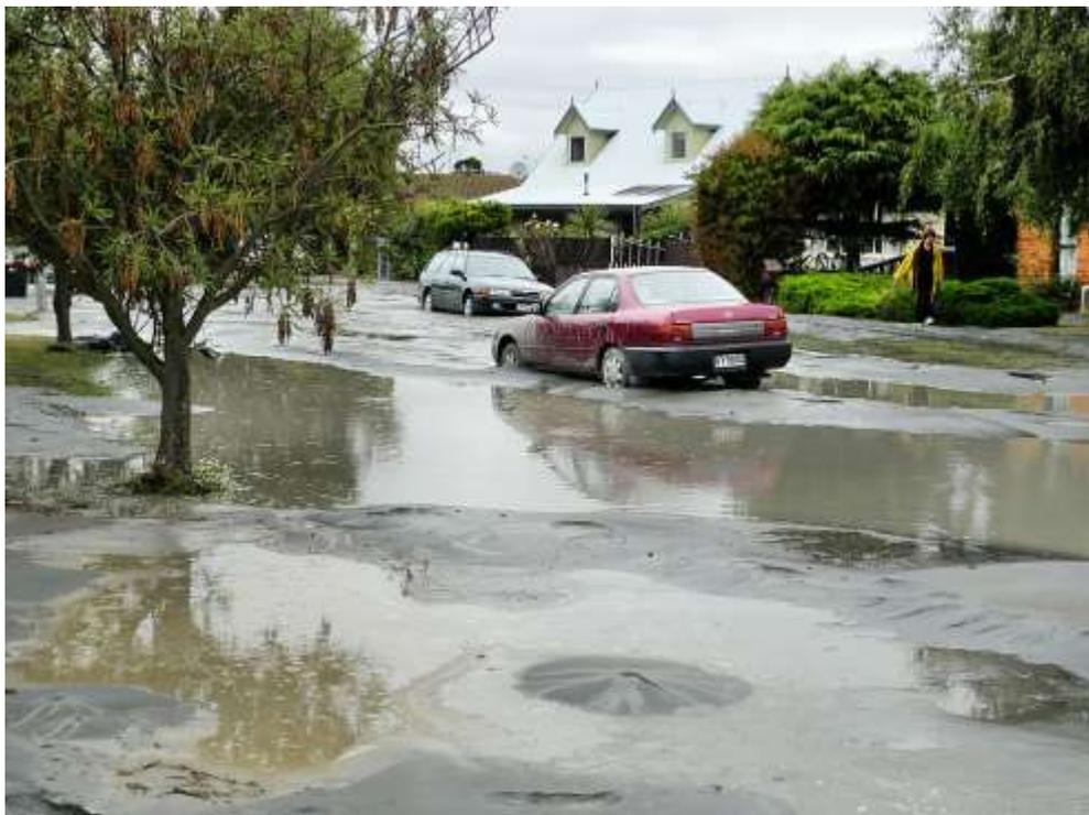
Figure 6. Liquefaction in Avonside following the February 21 Christchurch 2011 earthquake (photo by Martin Luff, Wikipedia Commons).
