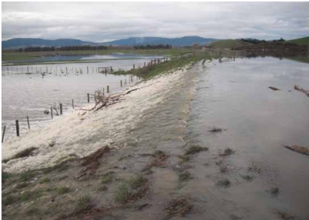
Figure 47. Overtopping of the Owhiro Stream into Area 17 (August 2012)
