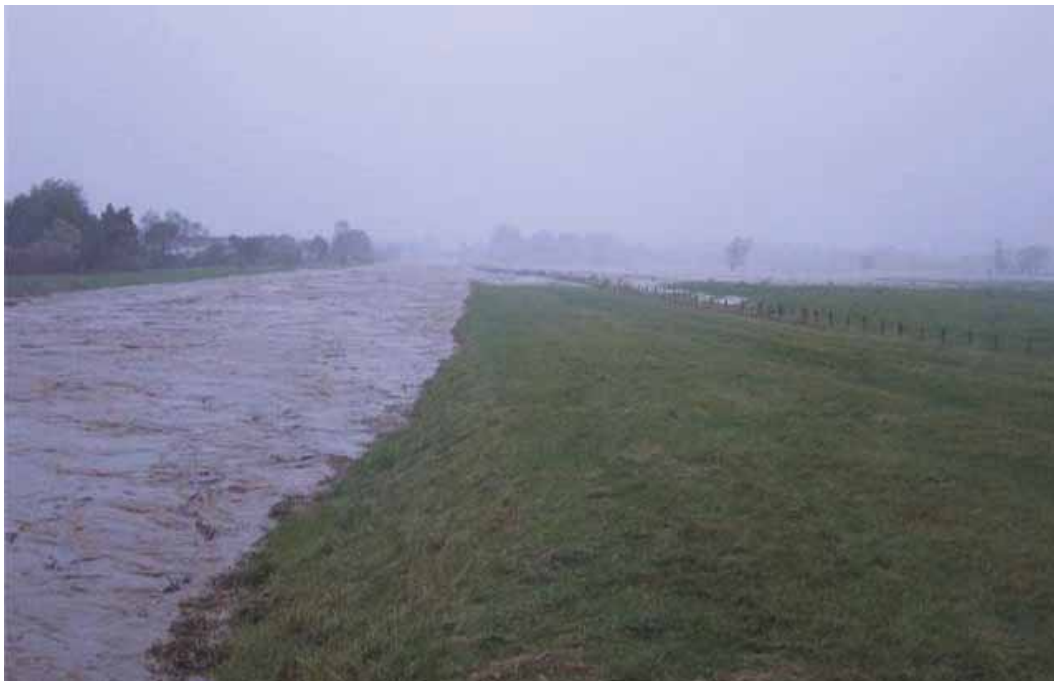
Figure 38. Silver Stream flows spilling over the Gordon Road spillway (April 2006)
