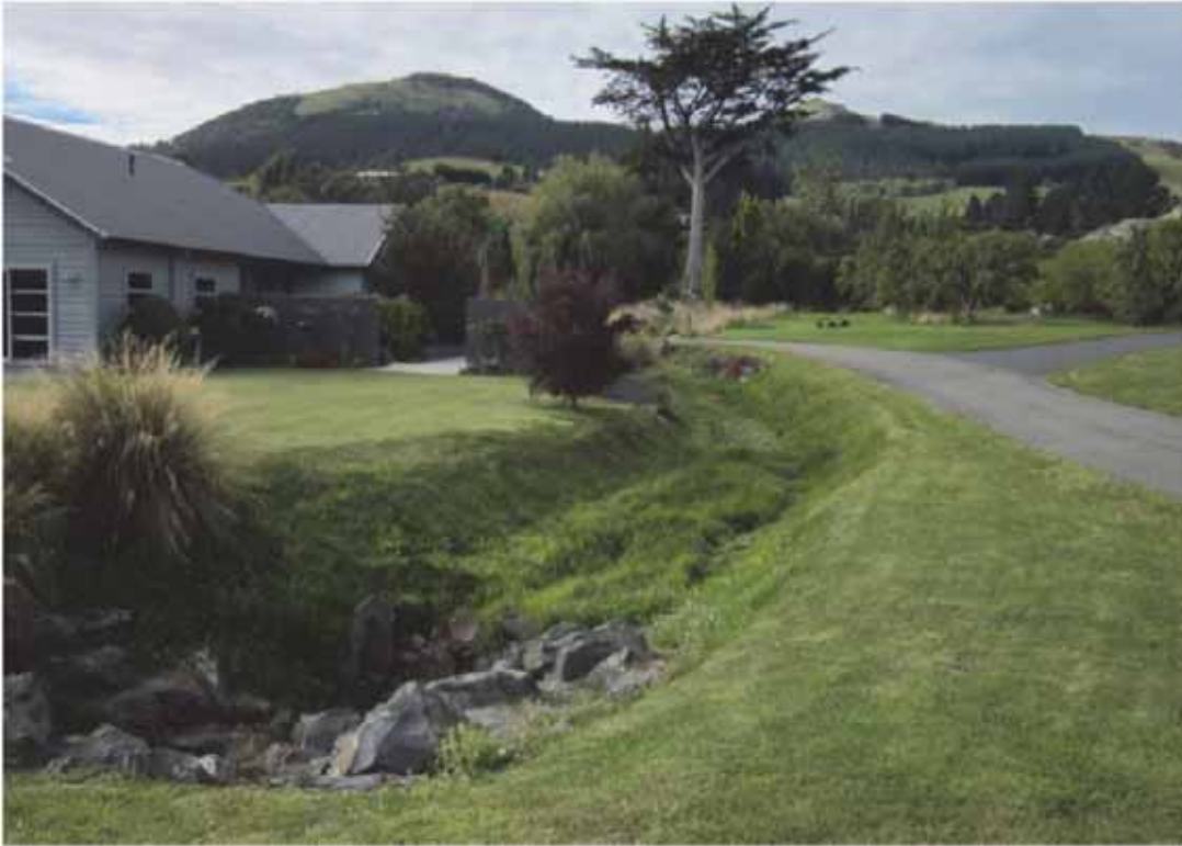
Figure 62. The engineered channel of Jaffray Stream at Orchard Grove, East Taieri. The head of its approximately 70ha catchment extends between Saddle Hill (left) and Jaffray Hill (right). (Photo: D. Barrell, 17 February 2014, GNS Science.)
