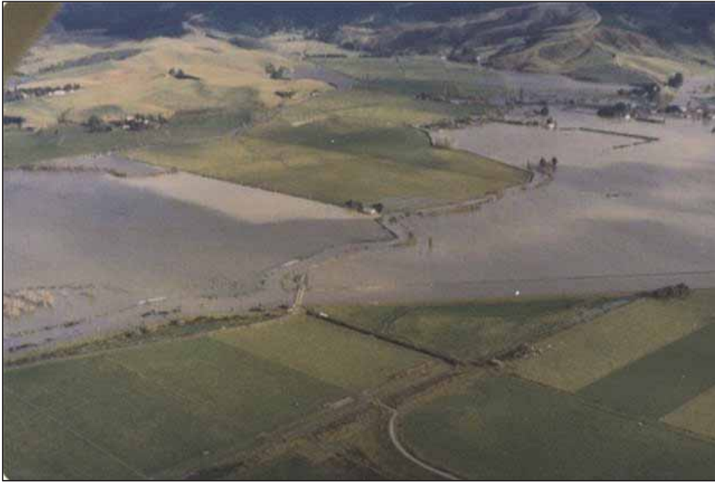
Figure 16. Aerial view of Waipori River No. 1 contour channel bridge, looking towards Berwick, May 1977. The photo was not necessarily taken at the peak of the flood.
