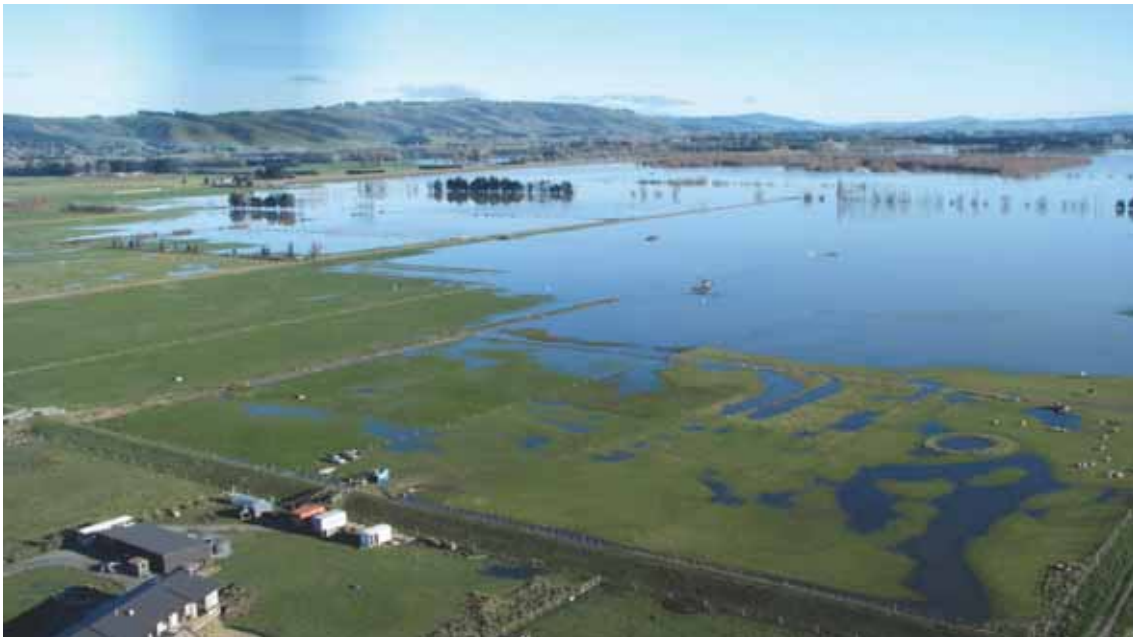
Figure 31. Water ponding in Area 12 on 31 May 2010. The Upper Pond cut-off bank is at the bottom of the image.
