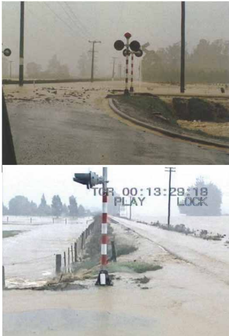
Figure 40. Water ponding behind the Taieri Gorge Railway, 26 April 2006
