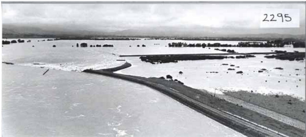
Figure 36. Breach of the northern section of the Area 13B ring bank during the December 1993 flood event. The location and direction of this photo are shown in Figure 33.
