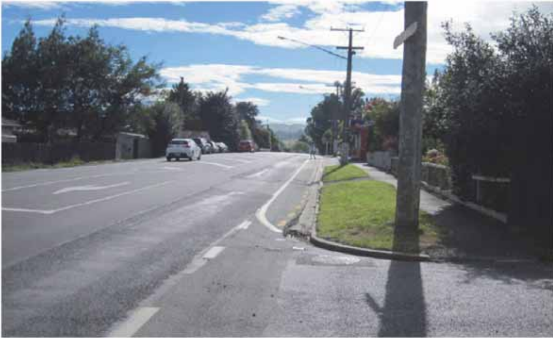
Figure 61. A view northeast along SH1 at East Taieri township, showing the fan of Jaffray Stream. The road rises over the fan axis, and Jaffray Stream is conveyed in a culvert at the point where the road goes out of sight. If the culvert were to become blocked by debris during a major rainstorm, there is potential for flooding and sedimentation on the fan surface. (Photo: D. Barrell, 17 February 2014, GNS Science.)
