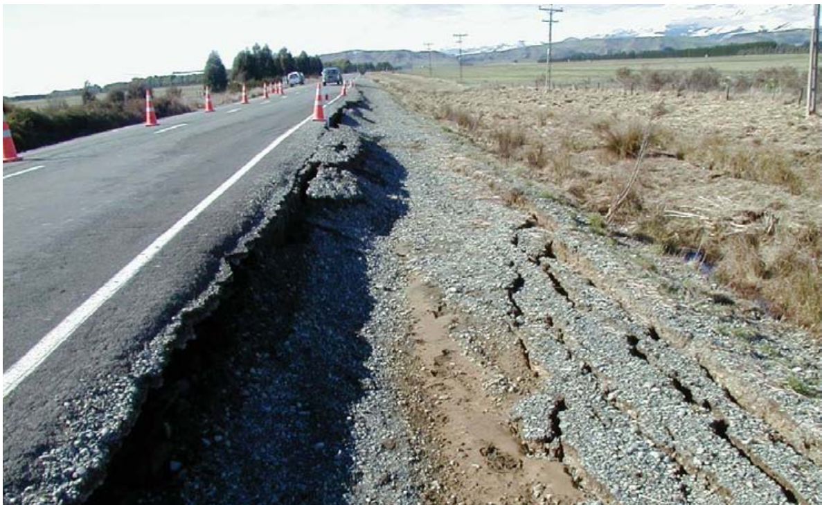
Figure 8 Damage to Hillside Road, Manapouri, Southland, resulting from the 2003 Fiordland earthquake. The road is raised on an embankment. Disaggregation of the embankment fill by ground shaking has caused a lateral spreading failure of the margins of the embankment. The existence of the embankment reflects the soft and saturated nature of the ground here, which probably exacerbated the earthquake shaking and consequential damage to the road. Photo: R Cook.
