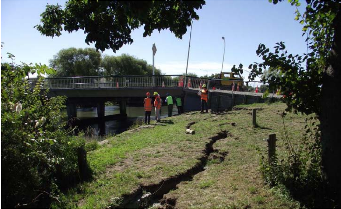
Figure 7 Lateral spreading and damage to bridge abutments as a result of liquefaction, Christchurch, February 2011. Photo: R.D. Beetham, GNS Science.
