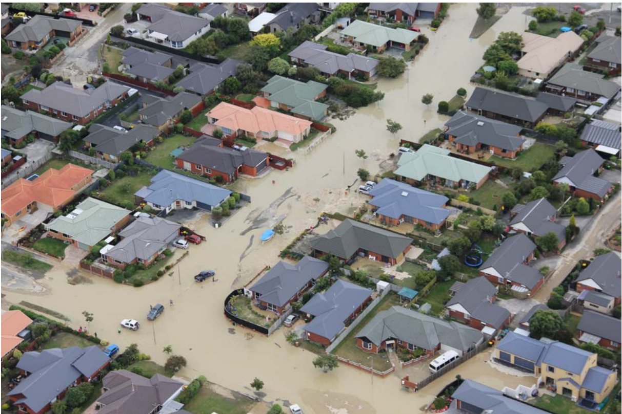
Figure 5 Extensive and severe liquefaction, Christchurch 2011. (a) Significant amounts (0.5 m thick) of sediment were ejected to the surface. (b) The liquefaction process also involved the ejection of large volumes of water which caused flooding. Photos: R.D. Beetham, GNS Science.
