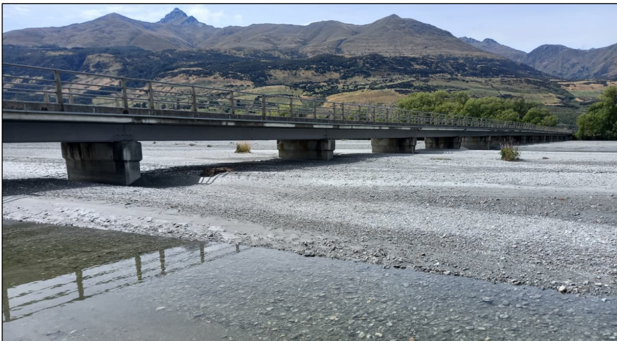
Figure 2.5: View of bed aggradation at the Rees River Bridge in January 2023
