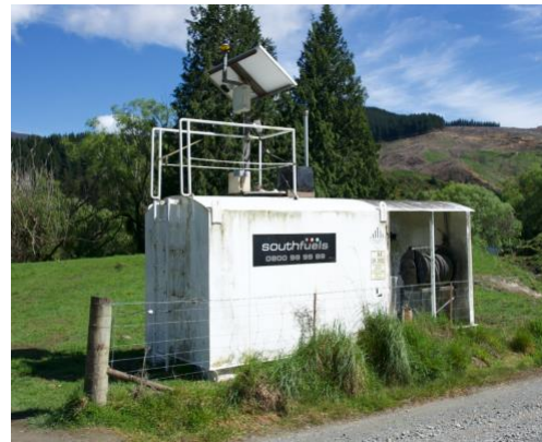
Photo 2. Existing fuel tank bundle at Beaumont site, 6 th Oct 2023.
