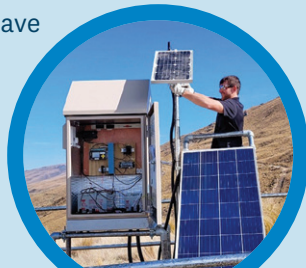
Brad Thomas (Environmental Technician) installing cabling for the new rain gauge
