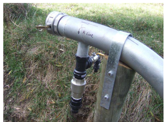
Outlet Source: ORC Inspection Sheets
