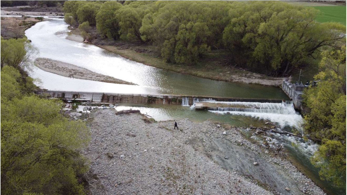
Figure 2 Photograph of the Omakau Irrigation Scheme main race intake on the Manuherikia River looking upstream.
