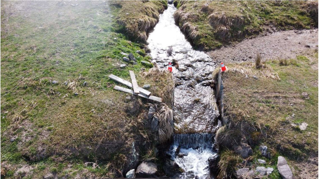
Figure 16 Photograph of the County race intake on Coal Creek looking upstream.
