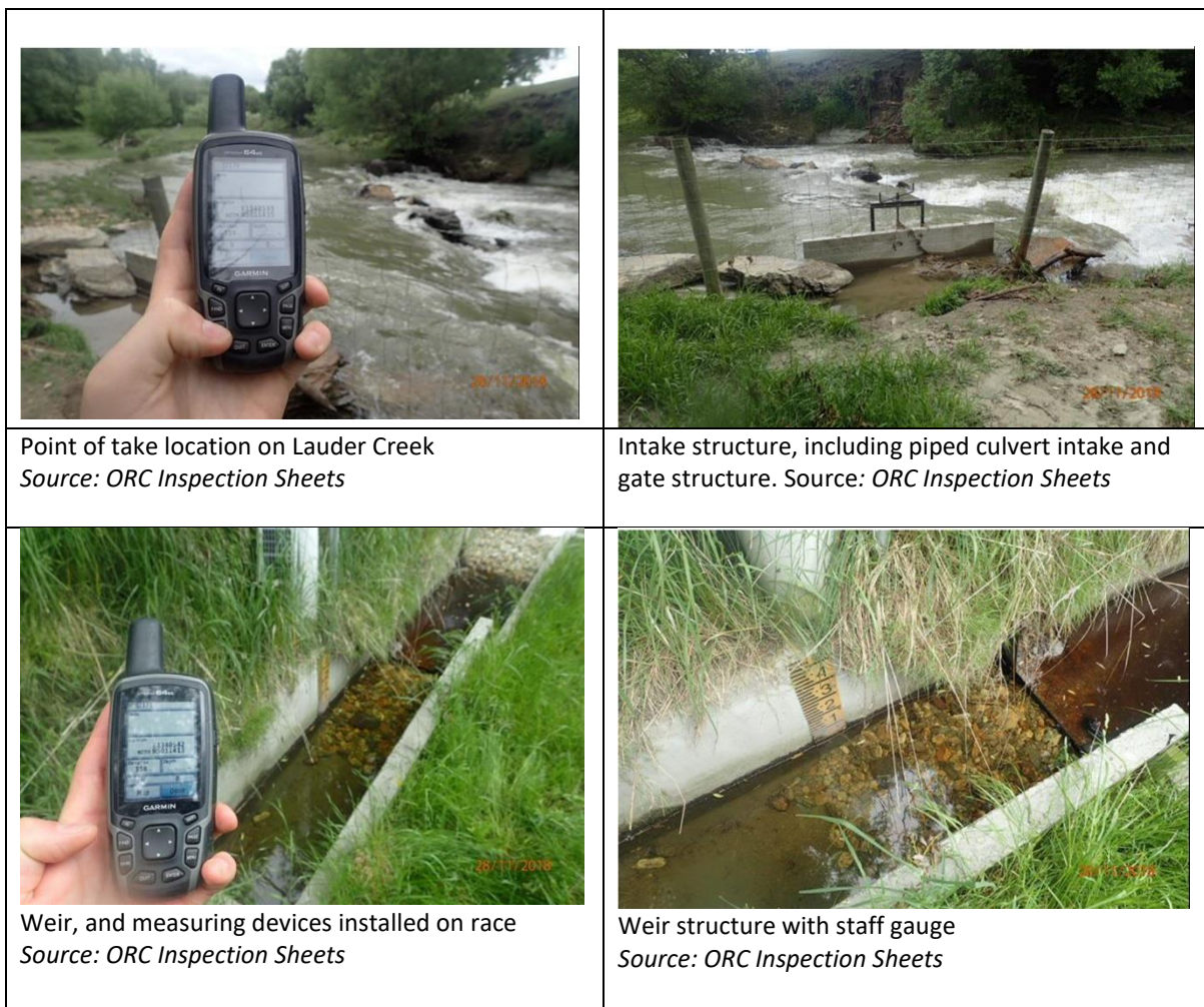
Figure 51 Photographs of intake and associated infrastructure under Permit 98122
