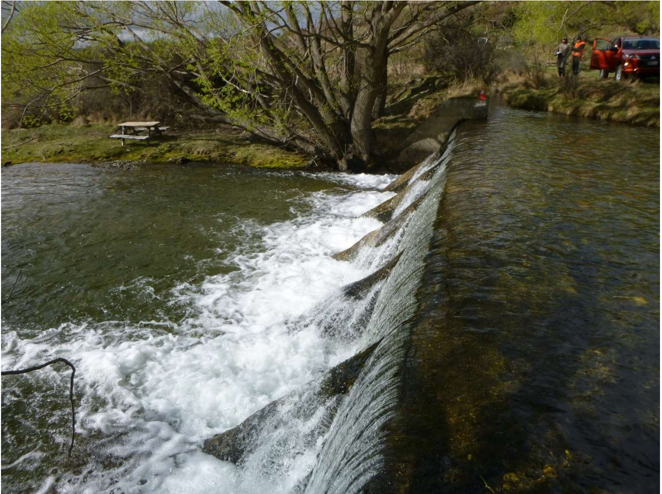
Figure 8 Photograph of the Lauder Creek race intake on Lauder Creek from the True Left bank.
