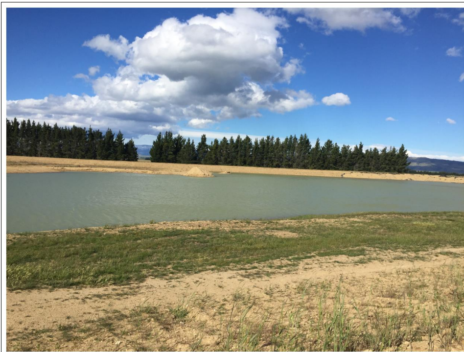
Figure 44 Photograph of Top Dam
