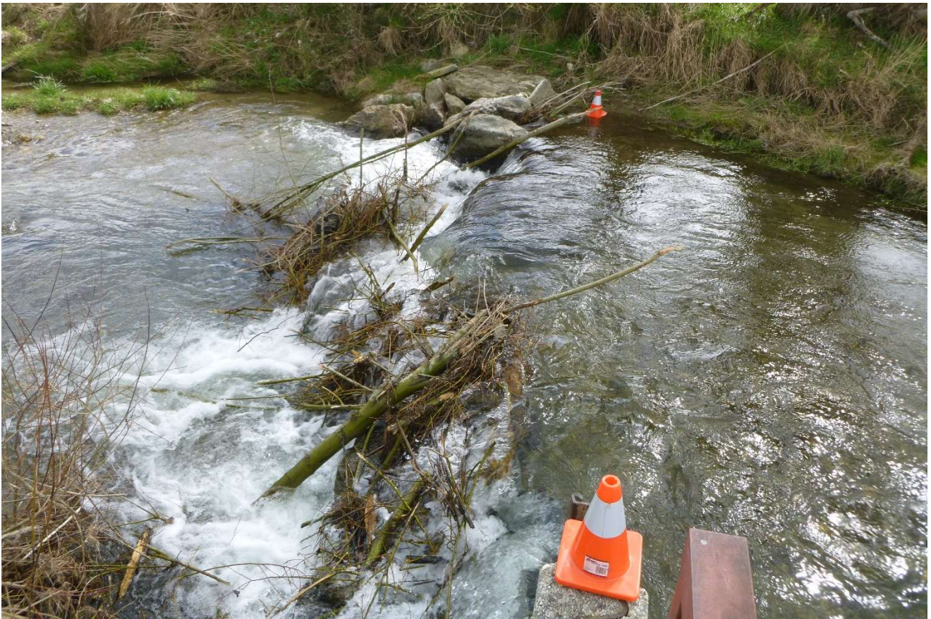
Figure 11 Photograph of the Clearwater race intake on Lauder Creek from the True Right bank.
