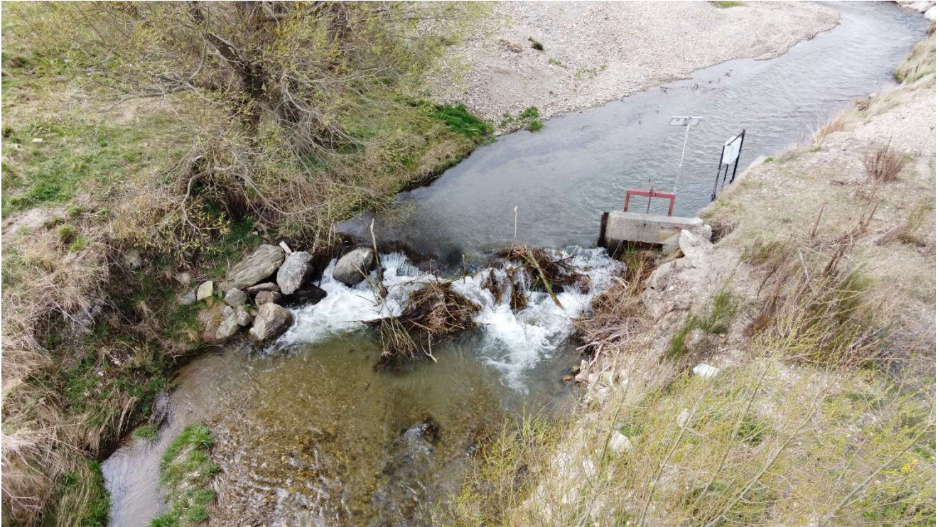
Figure 10 Photograph of the Clearwater race intake on Lauder Creek looking upstream.
