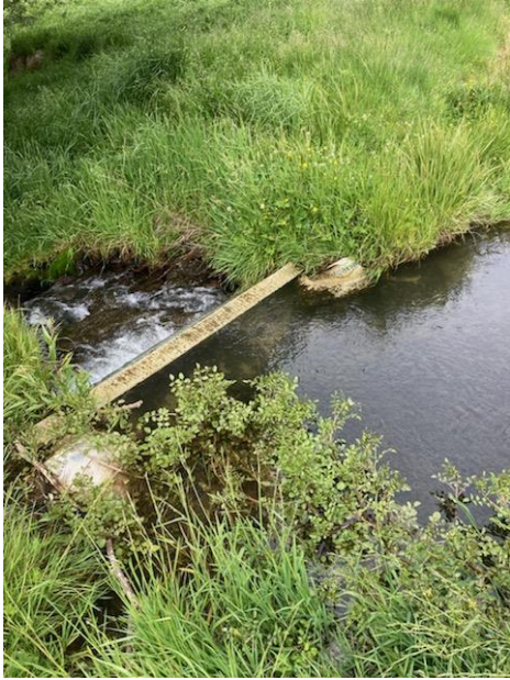
Millers Creek at intake, showing sandbags and board in the Creek guiding the flow
