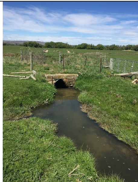
Photo showing culvert in the Creek with board gate structure. The raced intake is on the LHS in the mid ground.
