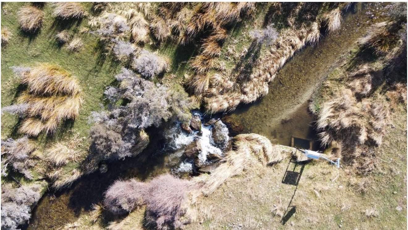
Figure 18 Aerial photograph of the County race intake on Middle (Buster) Creek.
