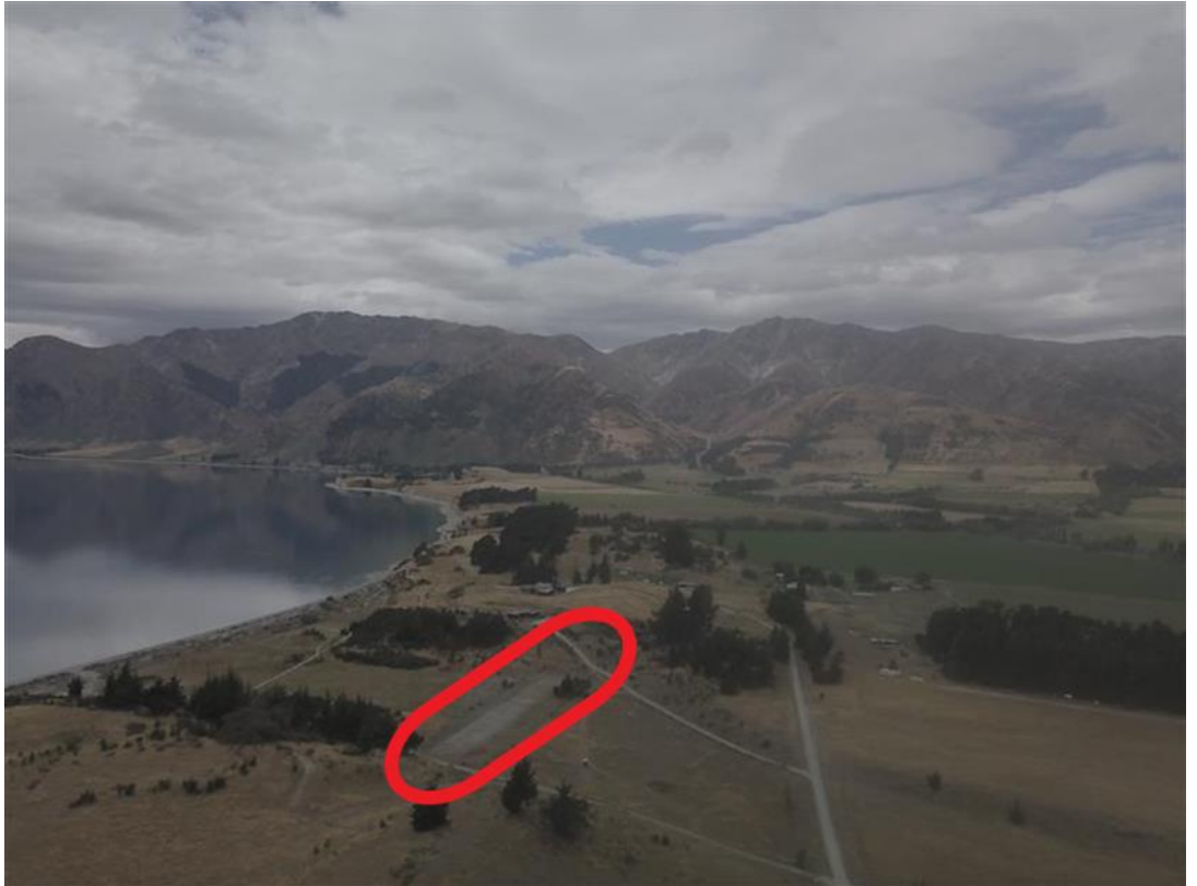
Figure 4: The Gladstone Gap Stopbank and Spillway
