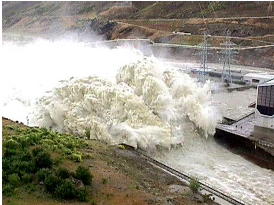
Photo 3: Clyde Dam spillway in 1999 flood
