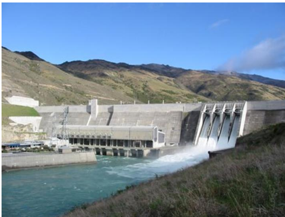
Figure 5: The Clyde Dam
