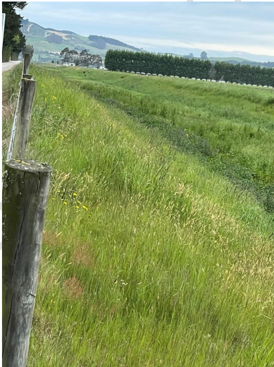
Figure 12: Henderson and Waikoura Creeks Floodway; viewed from opposite 550 Jardine Road, looking towards the south.
