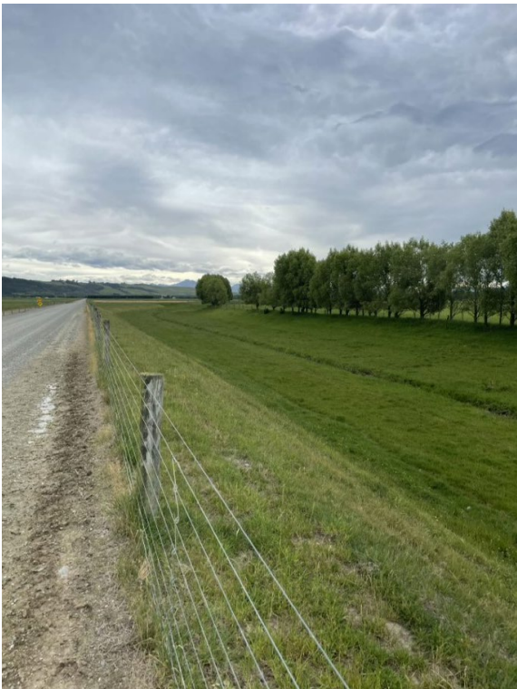
Figure 10: Henderson/Waikoura Floodway from Irvine Road (upstream)
