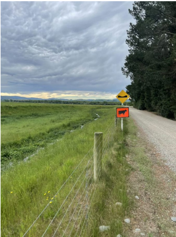
Figure 14: Henderson/Waikoura Floodway from Jardine Road (downstream)
