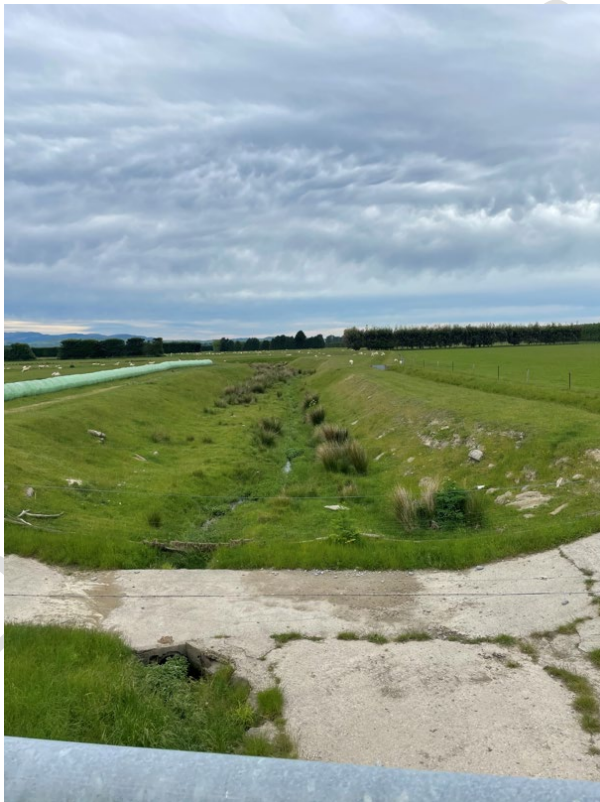
Figure 10: Waikoura Creek Floodway, viewed from State highway 83 towards the north east.
