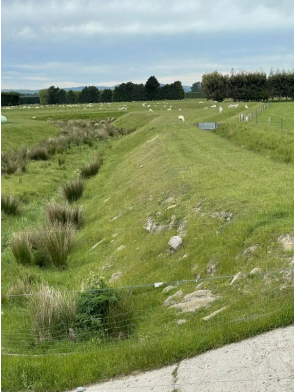
Figure 9: Waikoura Creek at State highway 83 (downstream). Note irrigation channel to the right of image
