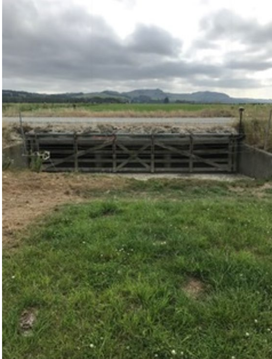
Figure 8: Eastern view of the Hilderthorpe Floodway Gray Road crossing
