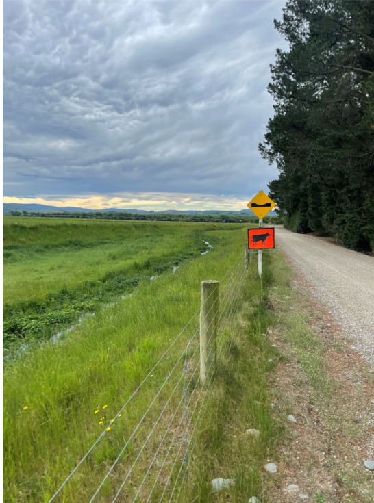
Figure 13: Henderson and Waikoura Creeks Floodway; viewed from opposite 550 Jardine Road, looking towards the north.
