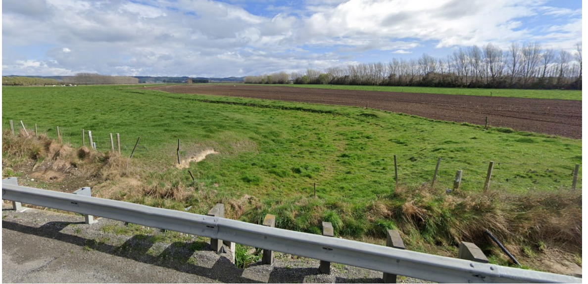
Figure 4: Hilderthorpe Floodway; view west from State highway 1 bridge
