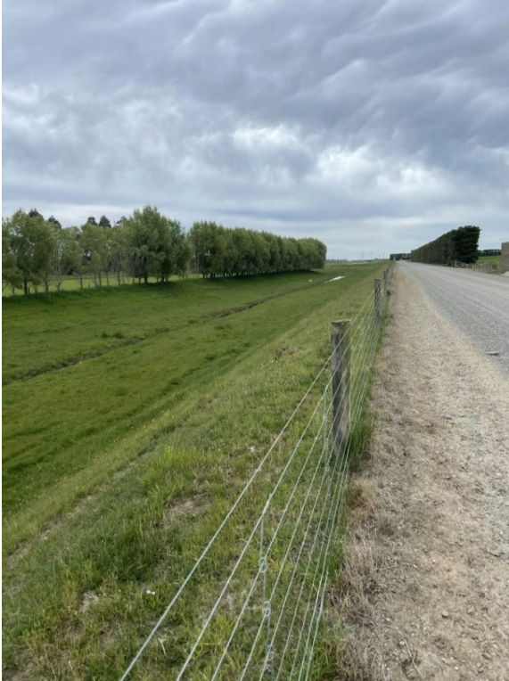
Figure 11: Henderson/Waikoura Floodway from Irvine Road (downstream)
