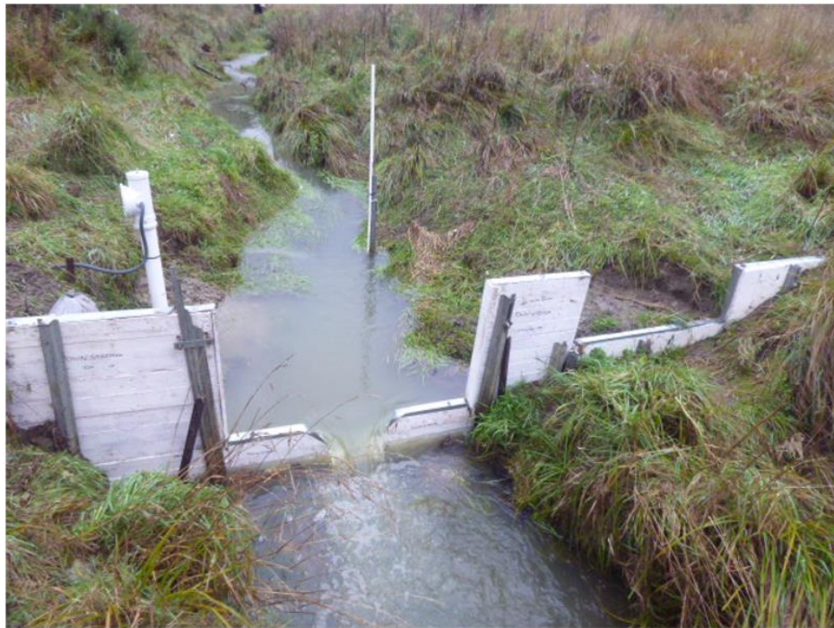
Photo 3: HopeHill Block Water Monitoring Unit. Photo by Matthew York.
