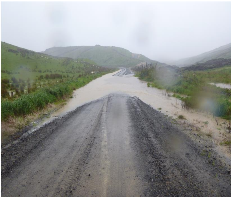
Photo 5. Flooding at McLaren Gully Road.
